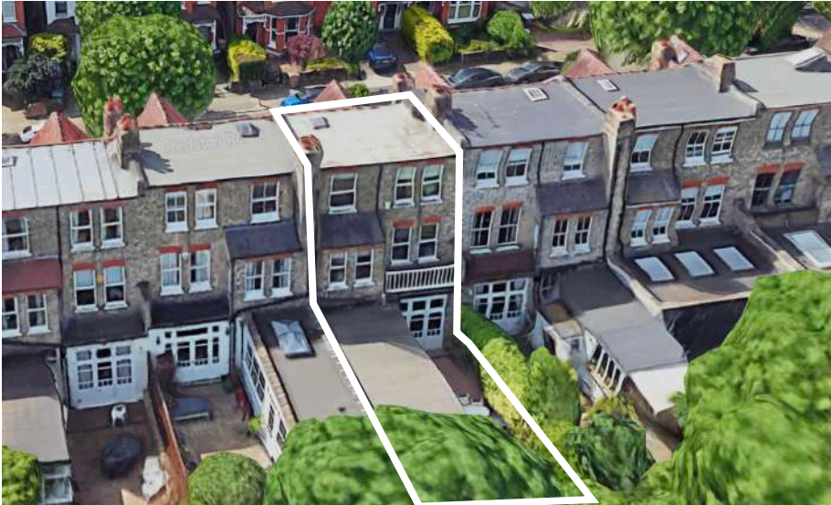
Fig 1.4 View of Rear No.93
