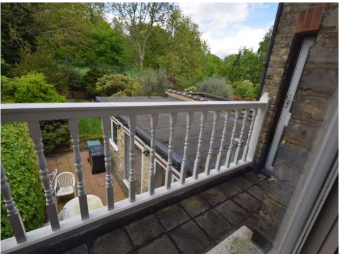
Fig 1.14 First Floor Juliette Balcony
