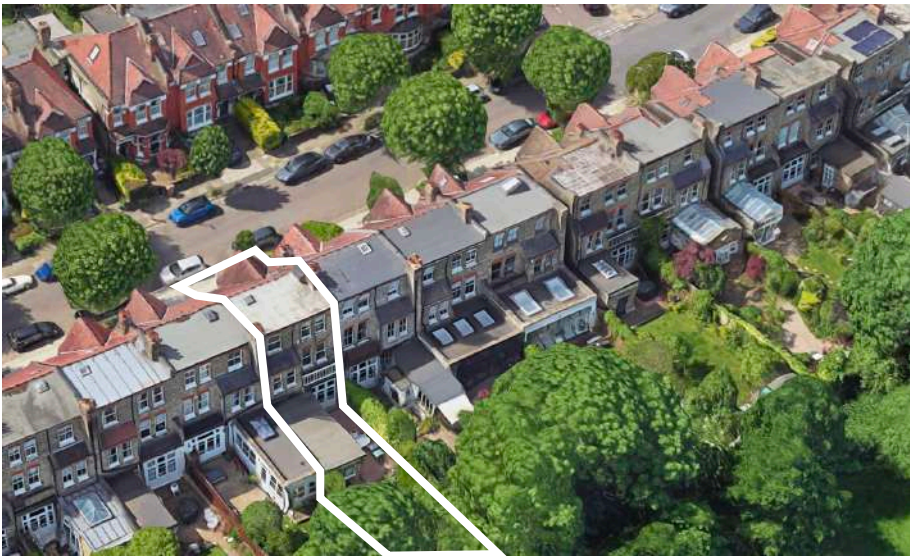
Fig 1.3 View of Rear No.93
