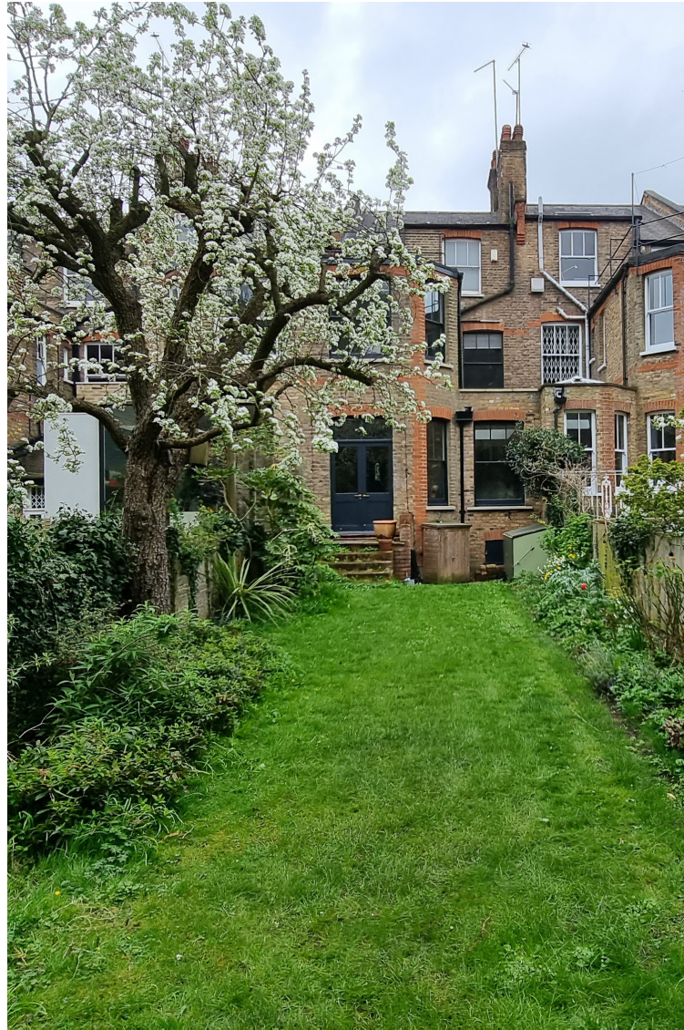
66 Priory Gardens | Rear Elevation
