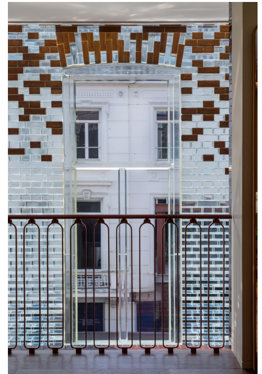
Balustrade At Hermes Store Amsterdam
