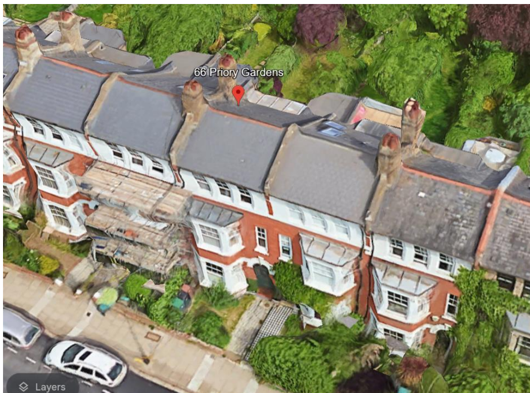
Figure 1 - Google Earth View of the property
