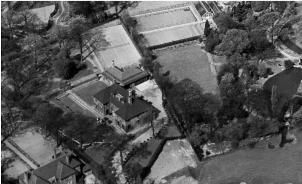
Figure 24: Sproughton in 1938 – with tennis court to the north west Historic England, EPW056796
