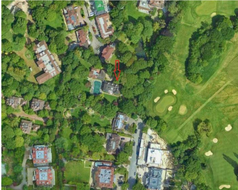
Figure 2: Sproughton, identified, with the Highgate Golf Course to the east, and mostly modern rooflines to north, west and south
