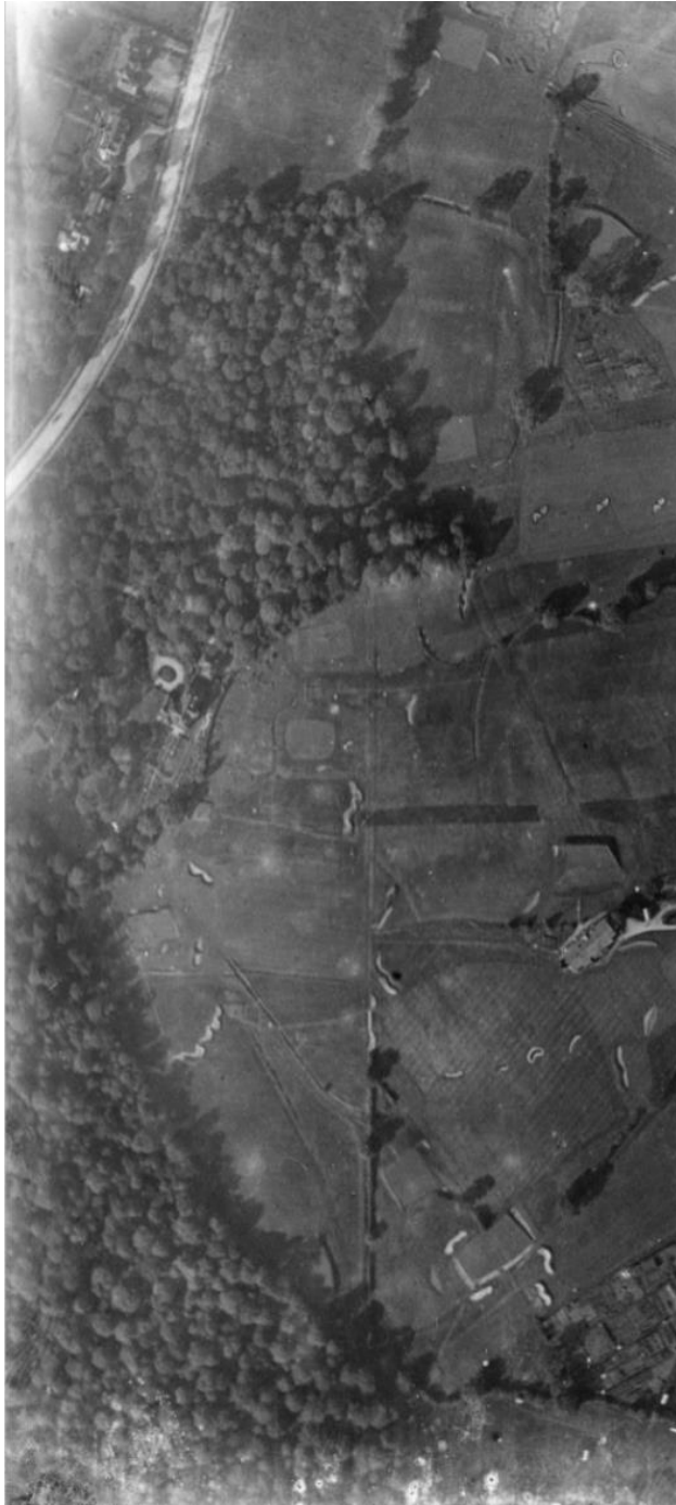
Figure 22: Aerial view taken in 1920: Courtenay Avenue is yet to be laid out, although the Golf Course (and Golf Club House) and The Bishop's Avenue, top left, are extant, with White Lodge already shown to the north east of the future site of Sproughton Historic England, EPW005115
