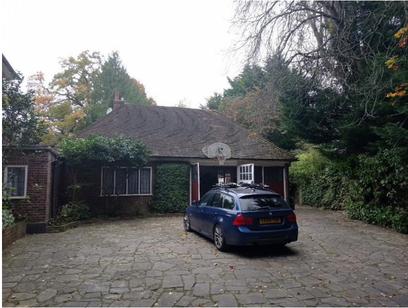
Figure 34: Garaging, since re-roofed and reconfigured
