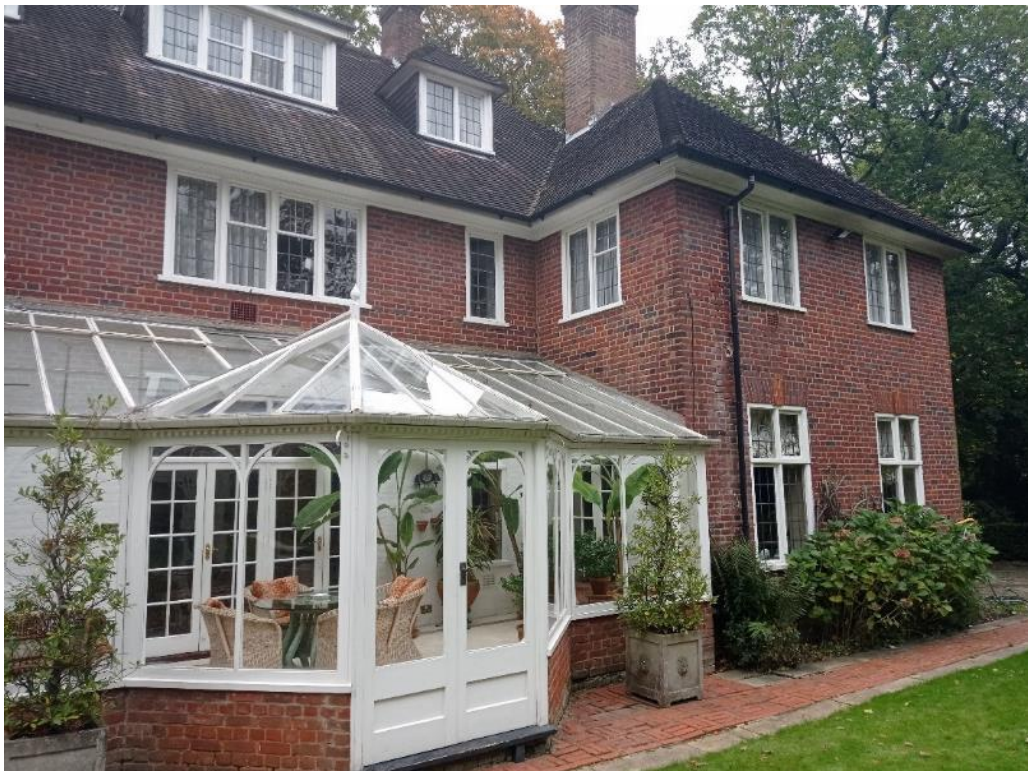
Figure 40: Rear elevation to Sproughton with late 20 th century conservatory
