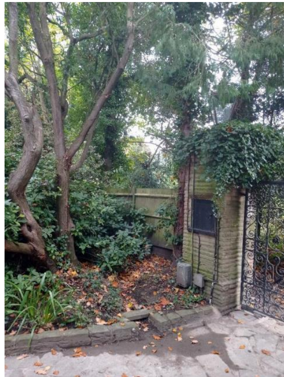
Figure 51: Entrance gate with pier, apparently later than the original marked
