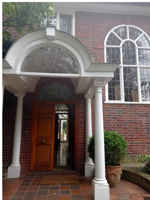
Figure 33: Late 20 th century portico with arched canopy, keystone motif, and fanlights
