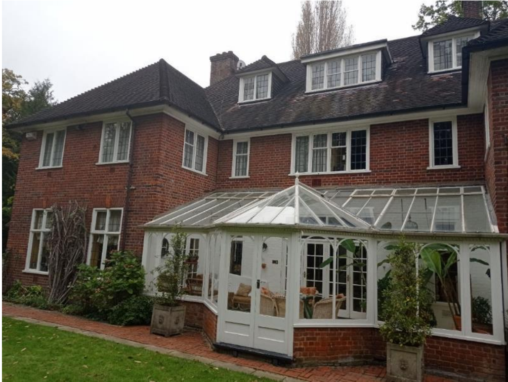
Figure 2: Rear elevation to Sproughton with late 20 th century conservatory
