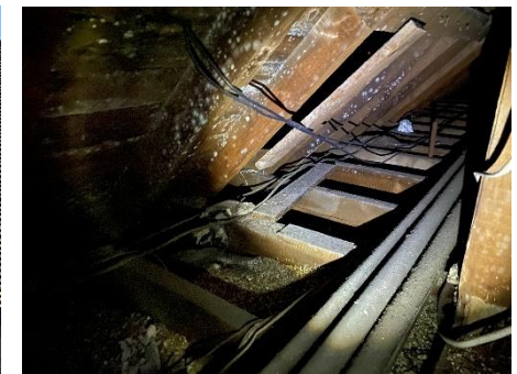
Figure 5: Internal loft void of main building
