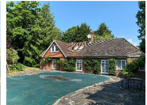
Figure 3: Adjoining building with hardstanding and swimming pool (covered)
