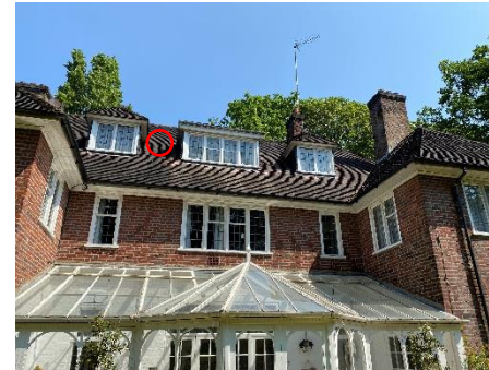
Figure 11: Western aspect of building. Red circle denotes the emergence location of an occasional day roost for common pipistrelle
