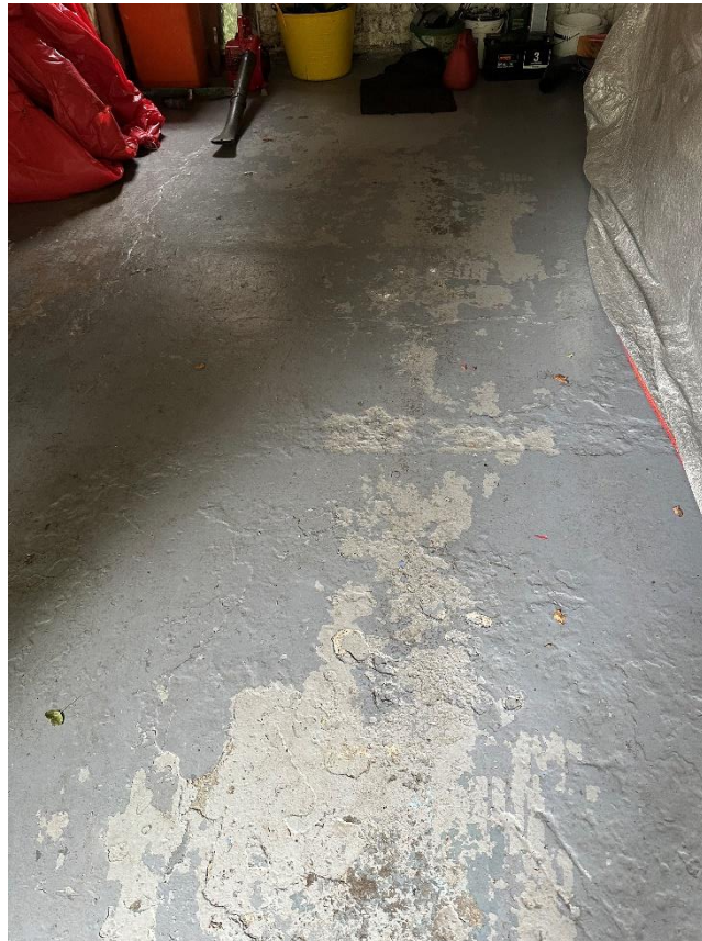
Figure 3: Major Concrete elements on site - Ground floor slab
