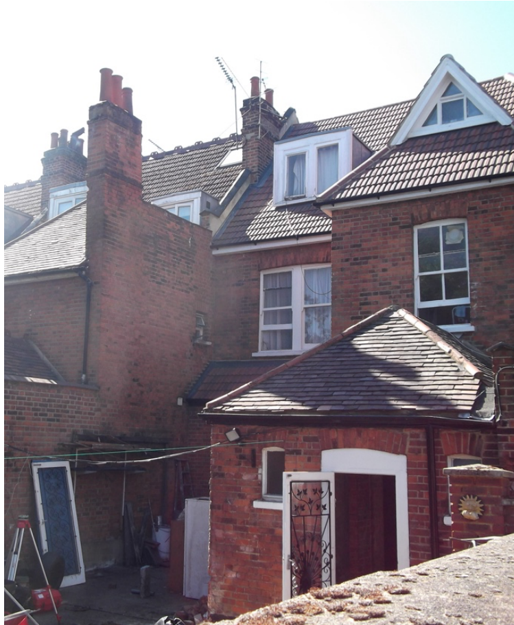
Fig 1. Above . Orange brick rear elevation of 46 Priory Road.
