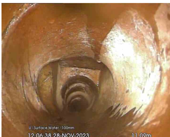
8-1-17A, 00:01:48, 11.09 m General remark, Approaching entry into manhole MH2
