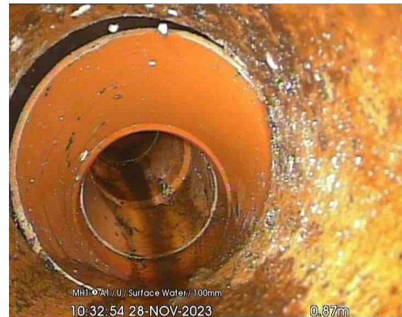
1-1-6A, 00:00:17, 0.87 m Open joint, medium
