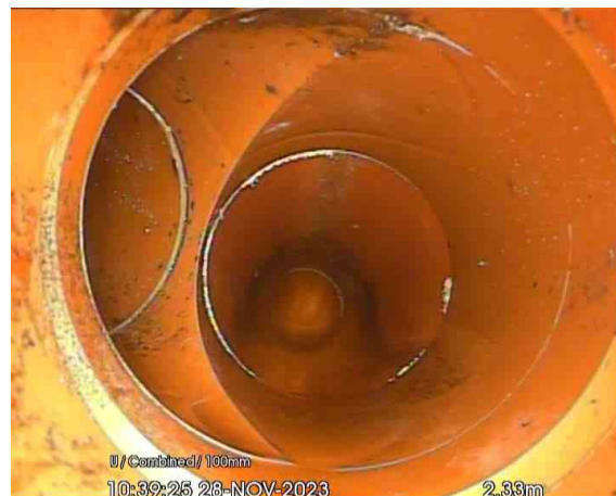
4-1-4A, 00:00:29, 2.33 m Junction at 9 o'clock, 100mm dia, A - not sourced
