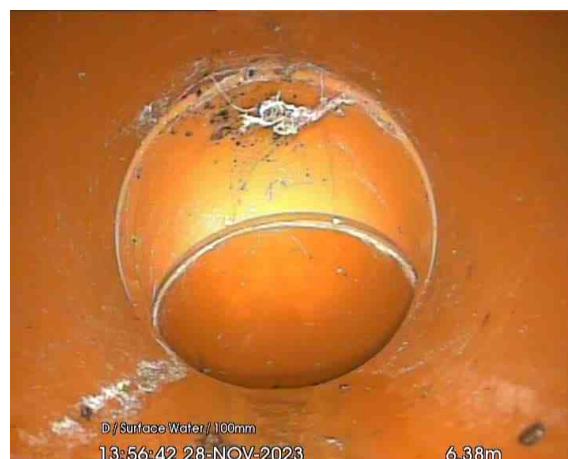
7-1-5A, 00:01:11, 6.38 m Line deviates down
