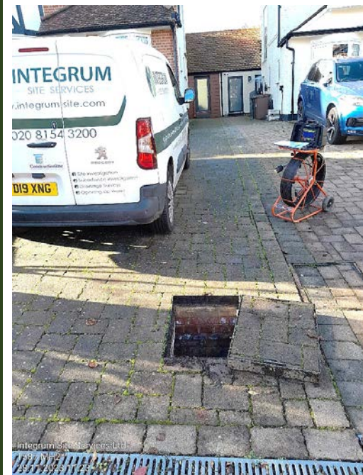
9. MH2 location overview
