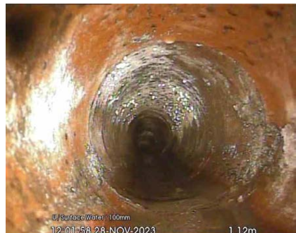
8-1-7A, 00:00:21, 1.12 m General remark, Camera enters line from SWG1 downstream
