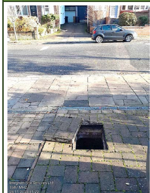
8. MH2 location overview
