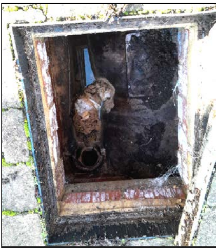
MH2: Depth 750mm (Interceptor Trap to FW line)
