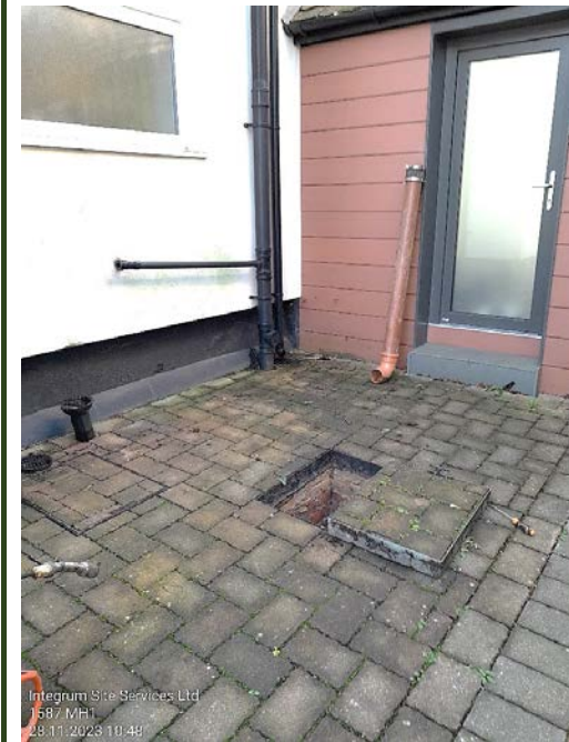
1. MH1 location overview
