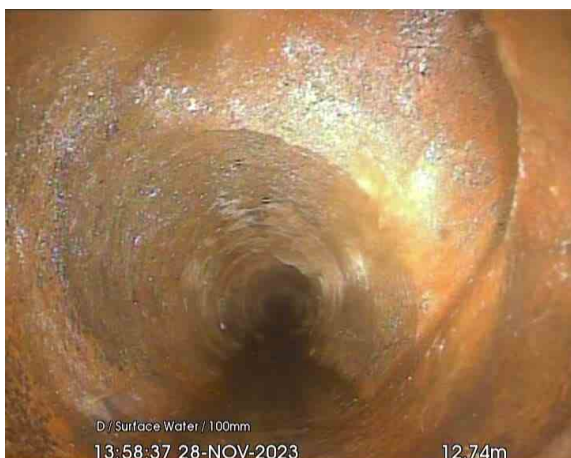
7-1-15A, 00:02:45, 12.74 m Junction at 1 o'clock, 100mm dia, G - not sourced / assumed original RWG2 junction
