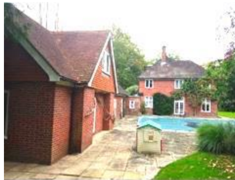
The Pool Facilities
