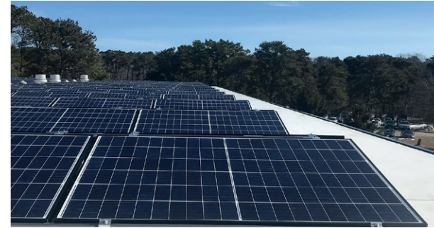
Figure 57: The large surface area of the roof provides enough space for a PV array to supply about 52,800 kWh per annum, to be used predominantly for lighting and appliances.
