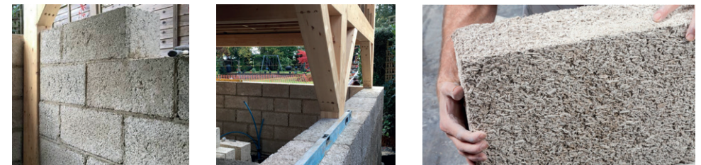
Figure 39: Hempcrete is a strong, lightweight and breathable building material made of hemp, lime and water. It is flame, water, mould and pest resistant and is known to last for hundreds of years. With excellent thermal properties, hempcrete has optimal moisture balance, and paired with the external lime render, allows the building to breathe and have a comfortable internal humidity level.
