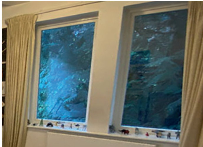
Room without a view. Overgrown tree branches cover windows
