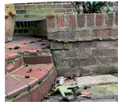
Cracking / Chipping
