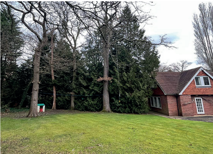
Pine Line encroaches House
