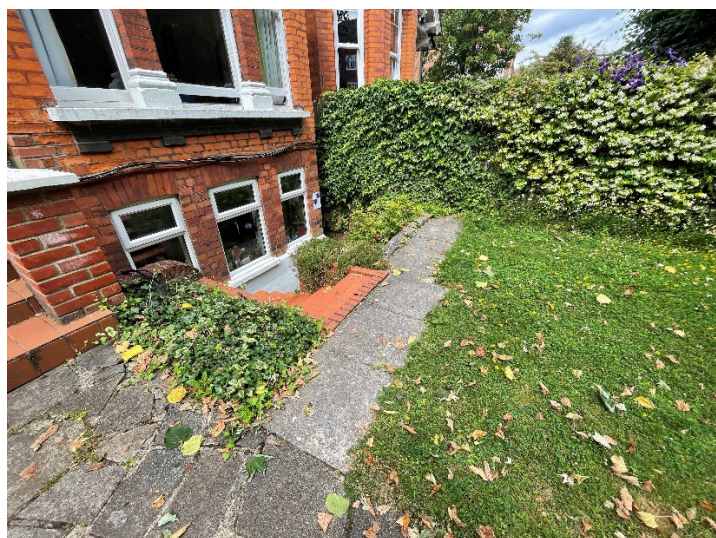
Open area to lower ground flat
