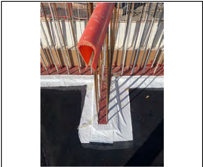
Successfully sealed perimeter beam
