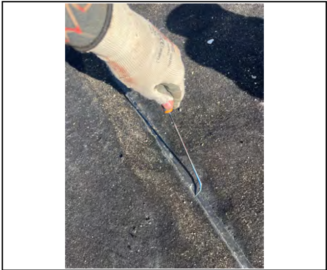
Pick and probe testing to welded
