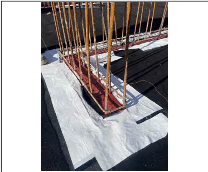
Successfully sealed pilecap detail.
