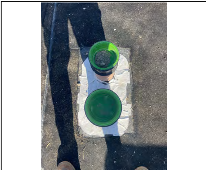
Successfully sealed pipe penetrations.
