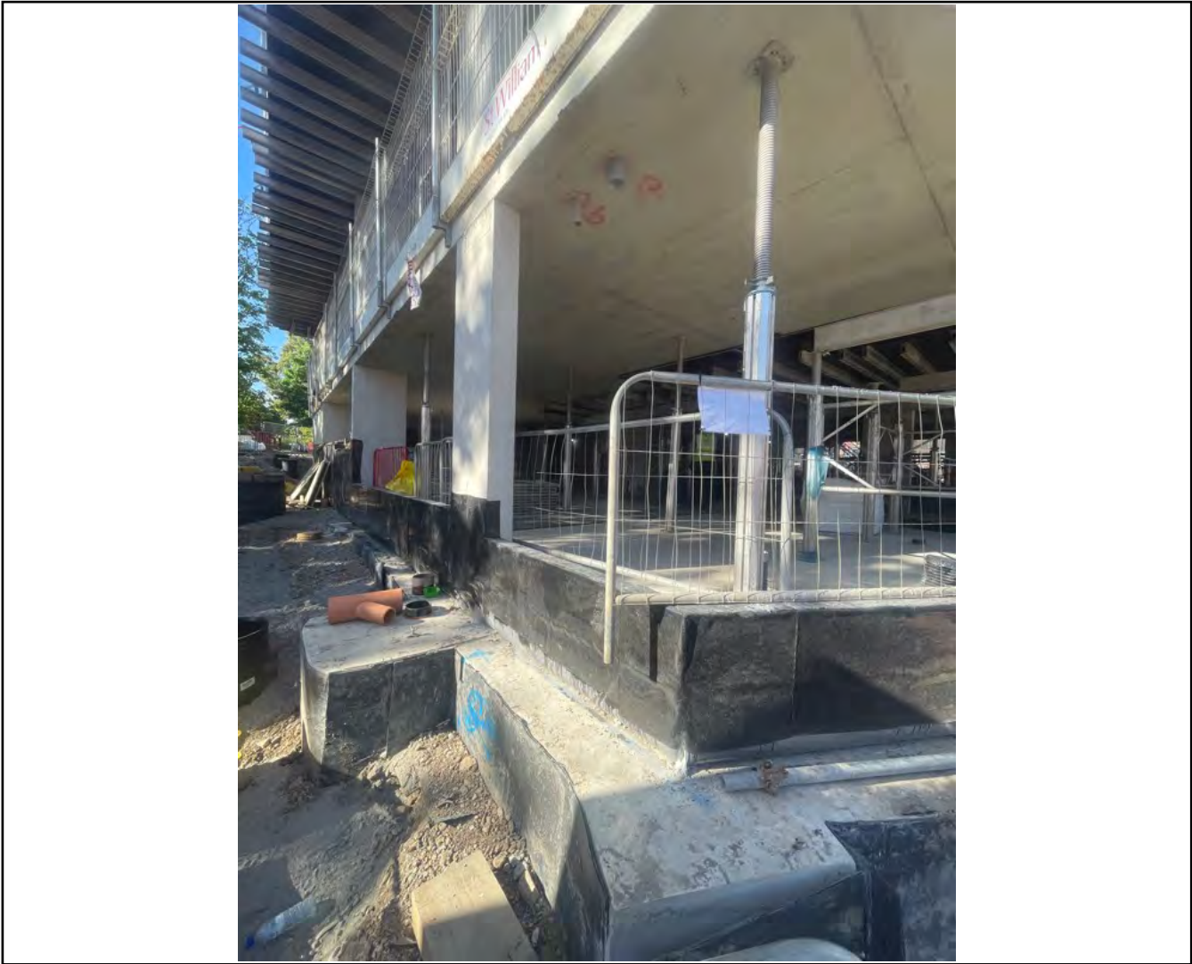
Overview photograph of the area verified during this visit.
