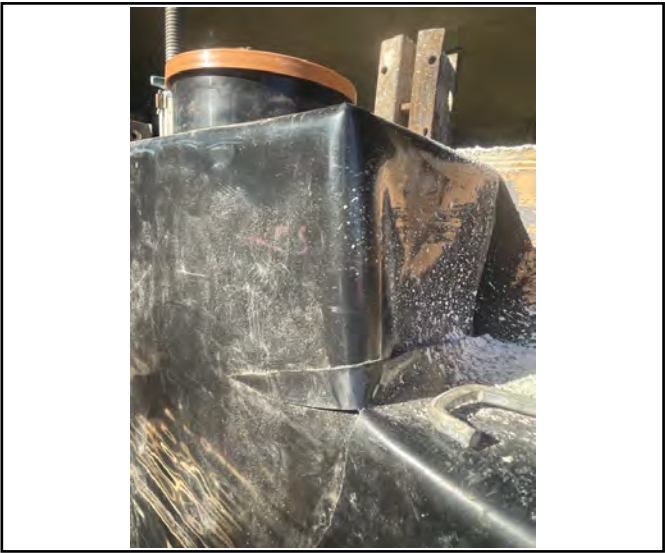
Intricate external corner detailing.
