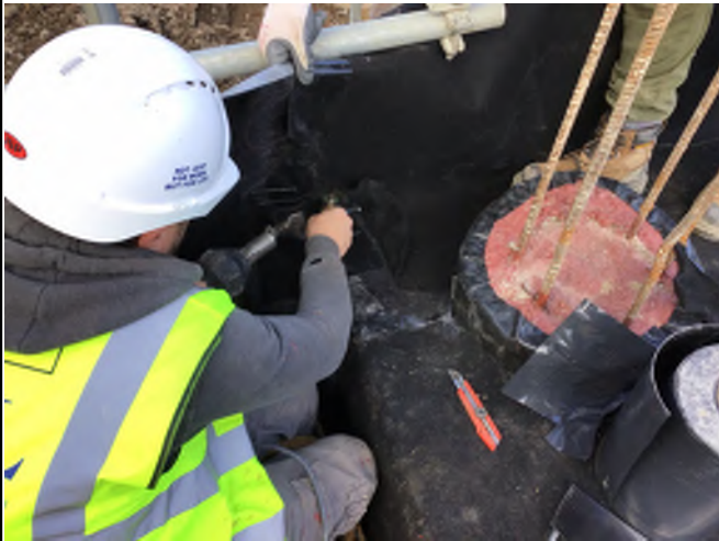
Last section of installation witnessed
