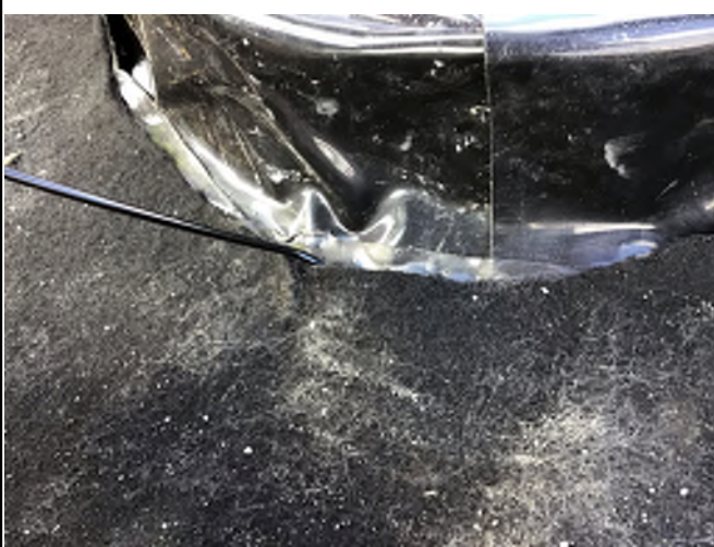
Pile heads fully sealed to Pudlo
