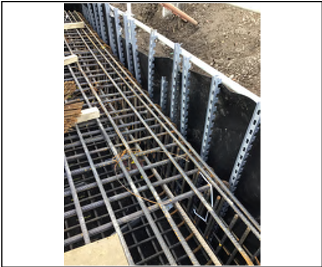
Tric trac spacers to vertical
