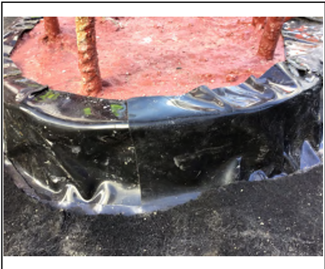
Pile head fully sealed
