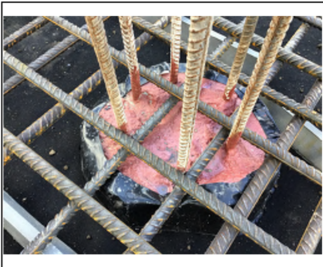
Pile heads all sealed
