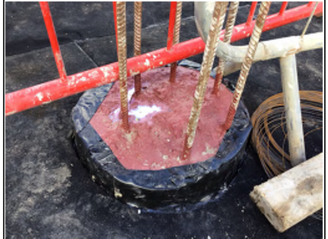
Pile heads fully sealed
