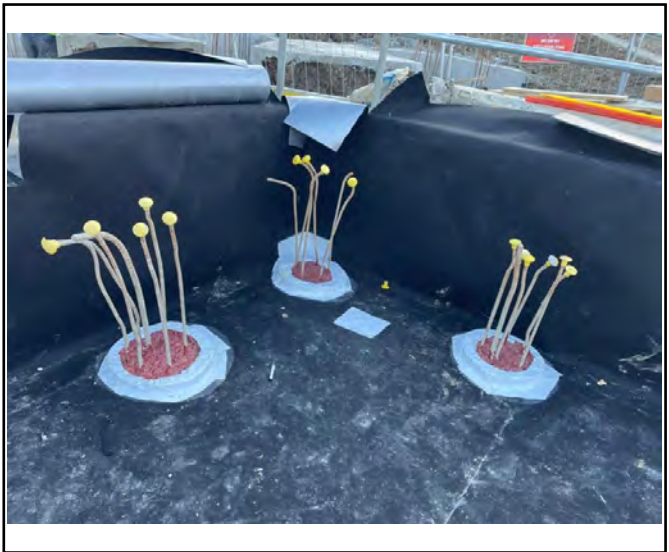
Overview photograph of the upper level.
