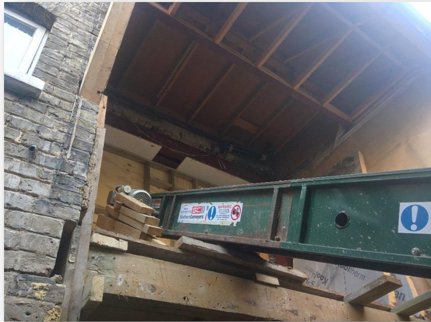
Conveyor to Remove Excavation Arisings
