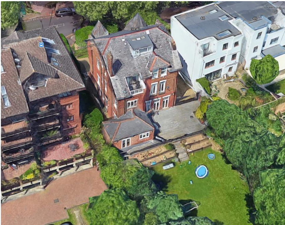
Figure 13: 3D view of the rear of the property, showing some localised modern intervention at roof level.
