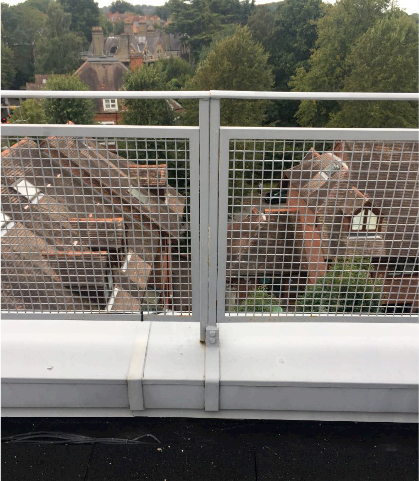
Existing guardings on South side (front) terrace
