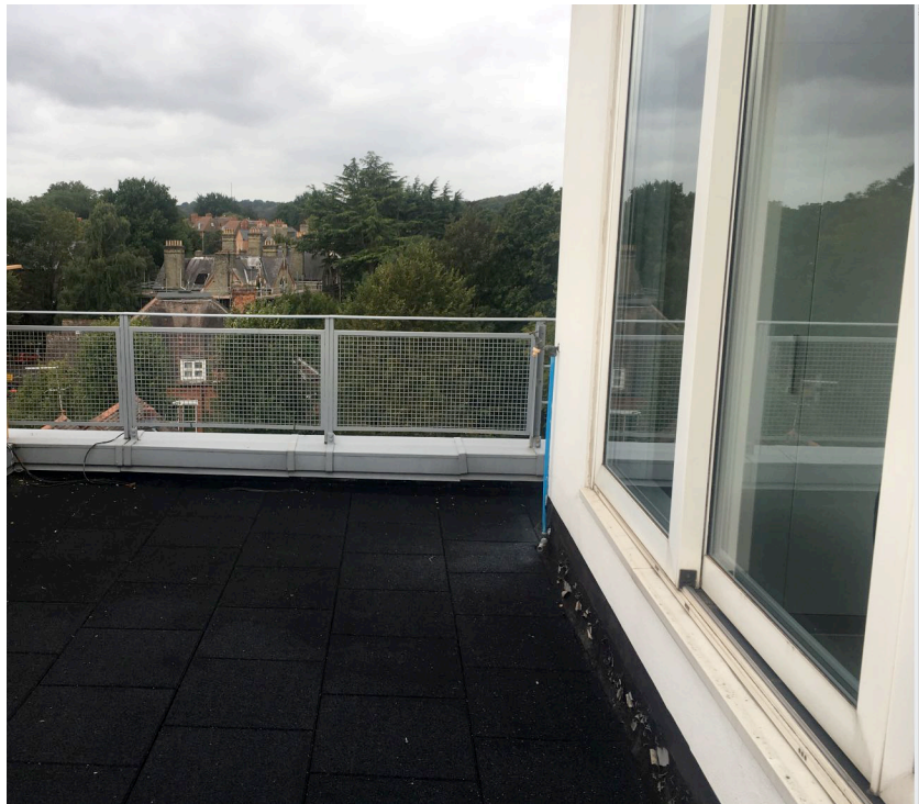
Existing guardings on West side of front terrace
