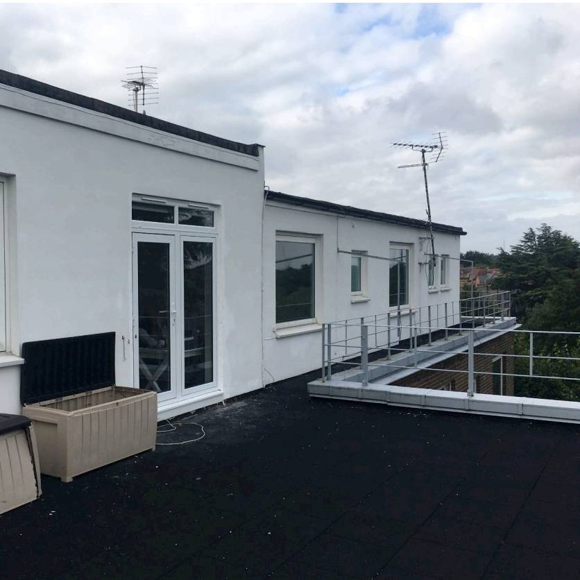
Existing guardings on rear terrace
