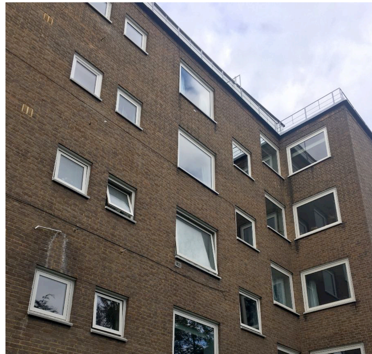
View of East facade
