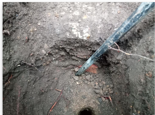
Fig 2.2: Trial Hole 2 Footing
