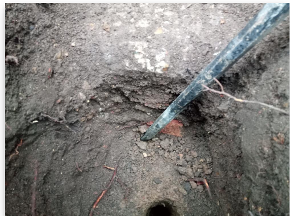
Fig 2.2: Trial Hole 2 Footing
