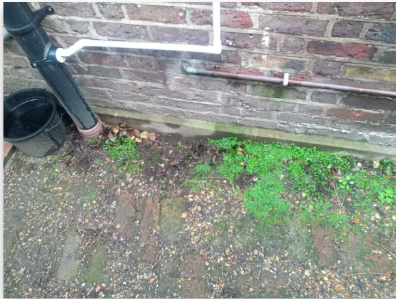
Fig 1.1: Trial Hole 1 Location
