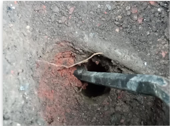
Fig 1.2: Trial Hole 1 Footing
