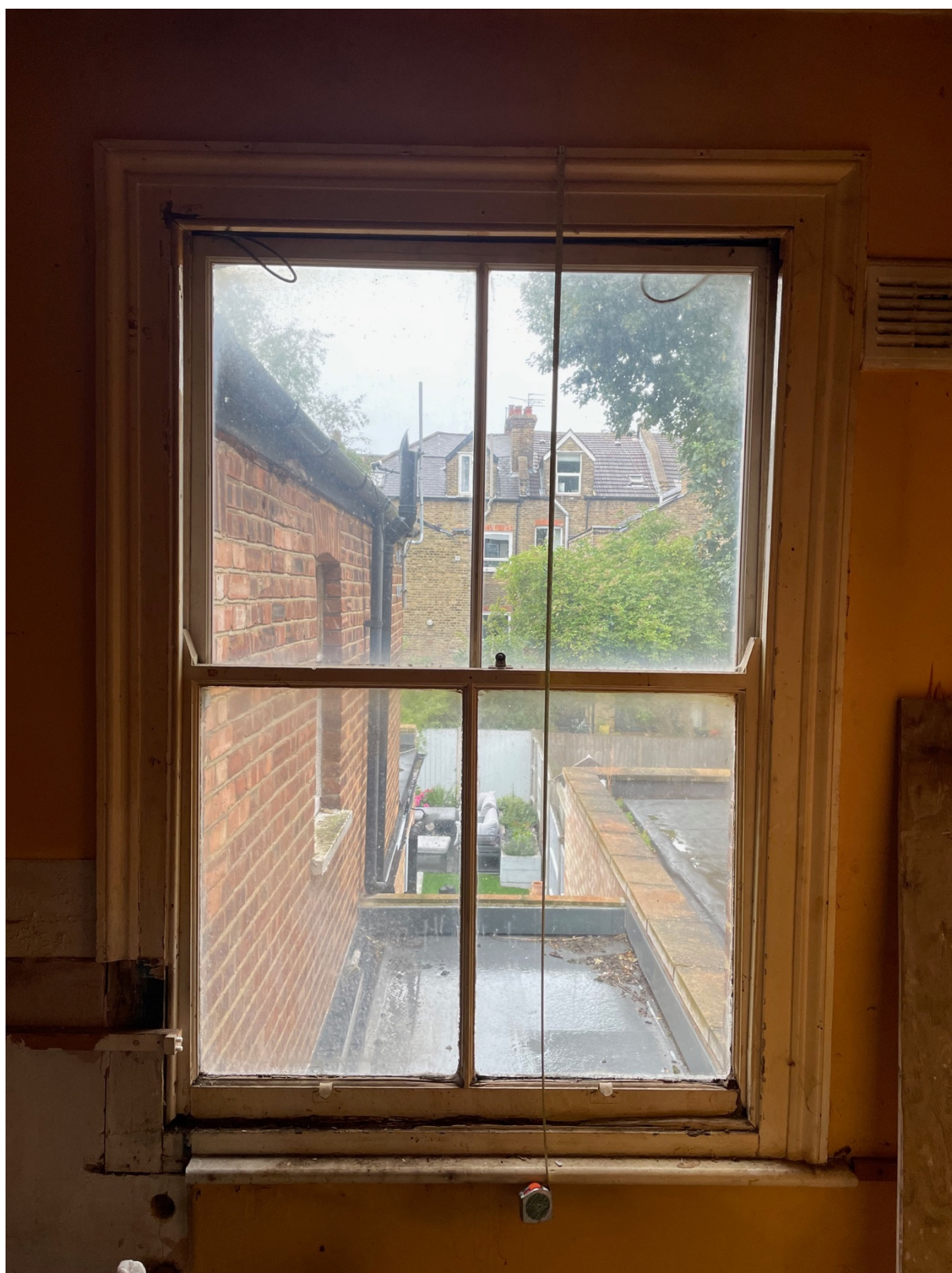
Single Sash Rear (Window D):
