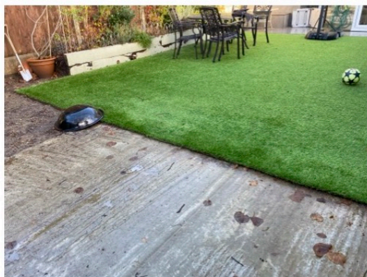
Existing ground slab to east of tree T1
