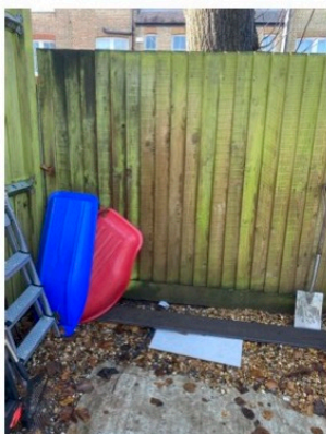
Boundary treatment - and existing utilities
