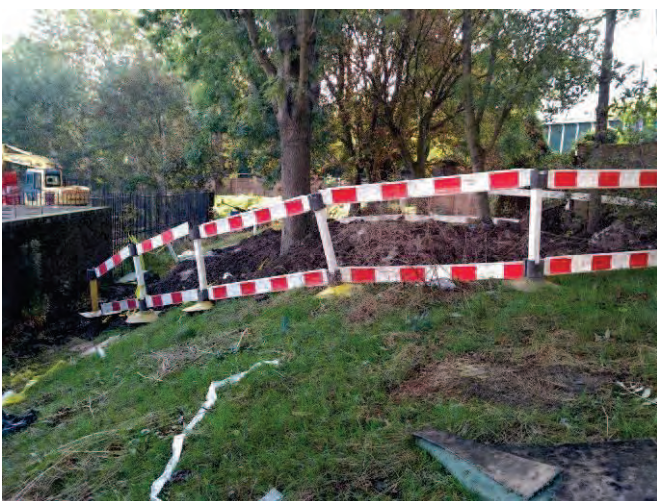
Plate 11: Area on the southwest of the site where the gas main has been repaired.
