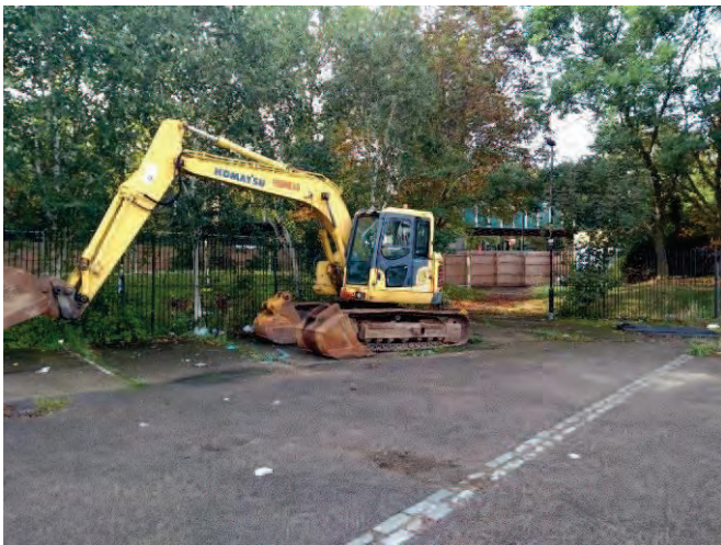
Plate 3: Southeast side of the carpark.
