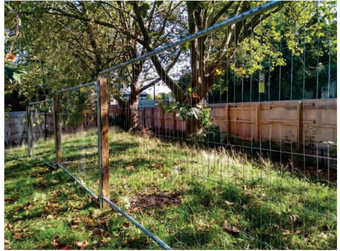
Plate 8: Tree Root Protection Area on the southeast of the site.
