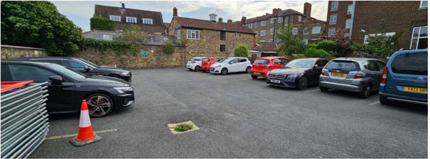
P4 Existing parking lot to north rear of development site
