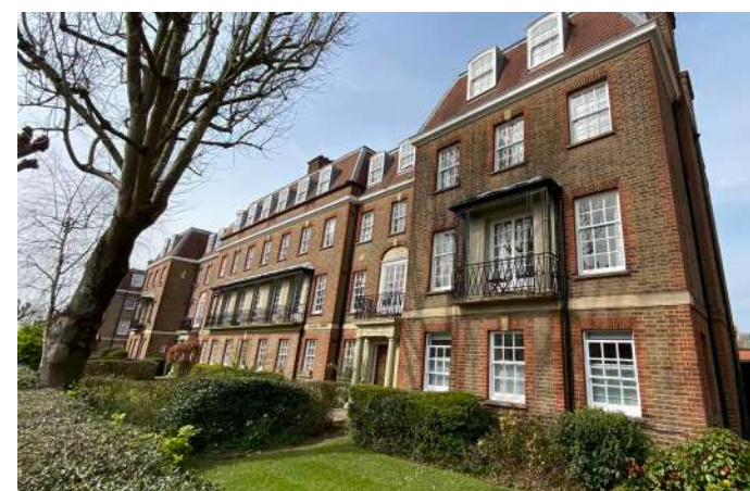
3. View of Twyford Court to the West of the site
