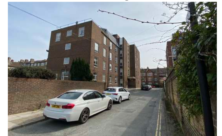
4. Rear of building from Spring Lane
