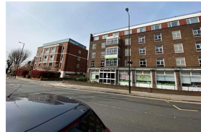
1. View of front of building showing Delphi Court to the West of the site
