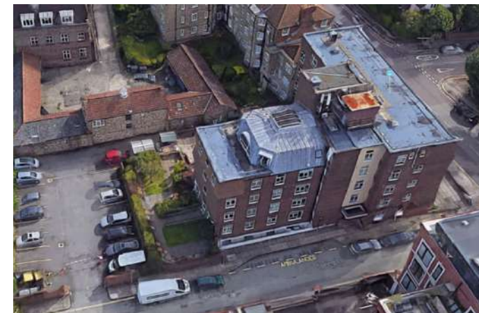
3. Aerial view of existing Care Home
