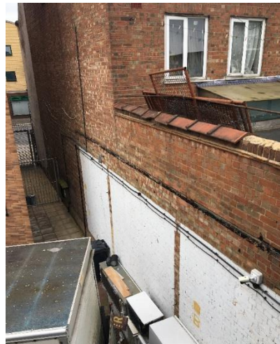
Pedestrian access from West Green Road
