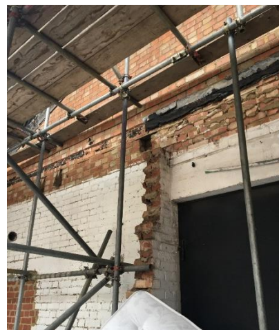
Existing condition of single skin brickwork on southern elevation
