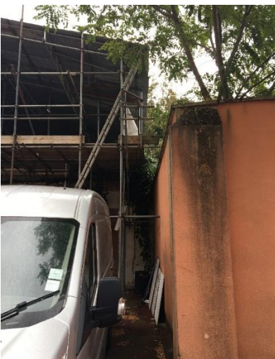
Gap between eastern boundary wall and existing warehouse wall
