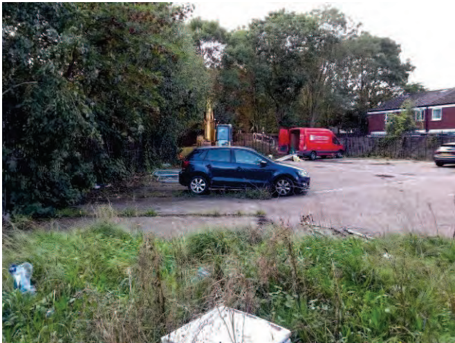
Plate 1: Looking south across the carpark on the north of the site.
