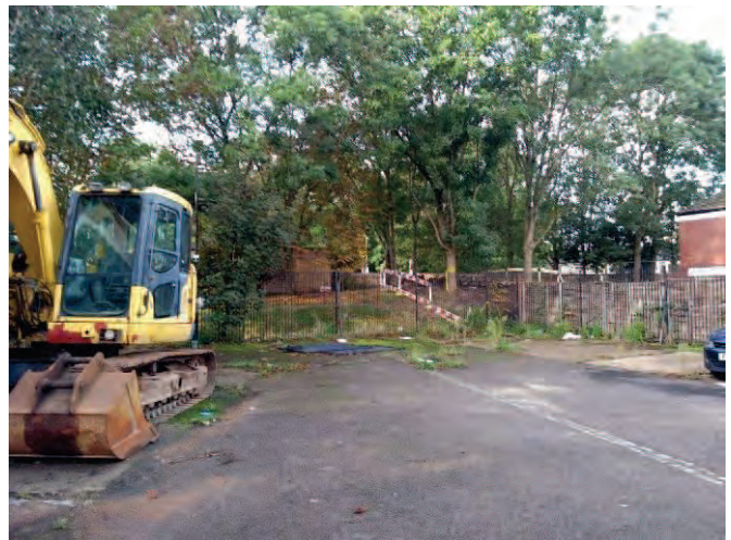
Plate 4: South side of the carpark.
