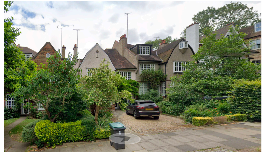
fig 4.2 Street view showing houses no 45 - 51
