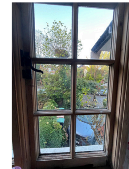
fig 3.5 Timber casement windows internal view
