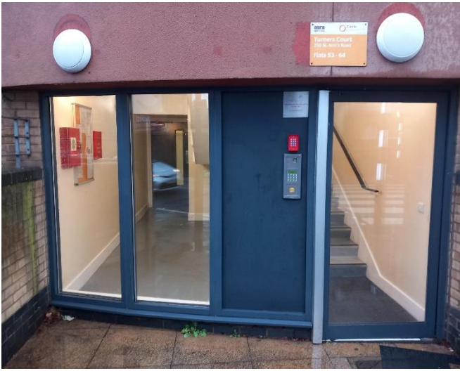
Block Entrance Door
