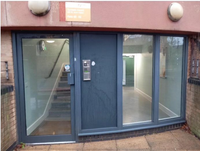
Block Entrance Door
