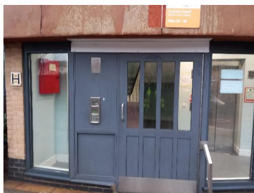
Example Communal Front Entrance Door
