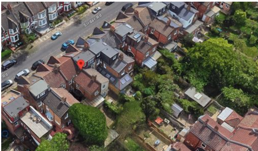
6. Rear view of the terrace showing wraparound extension at 23 Sirdar Road and other rear extensions
