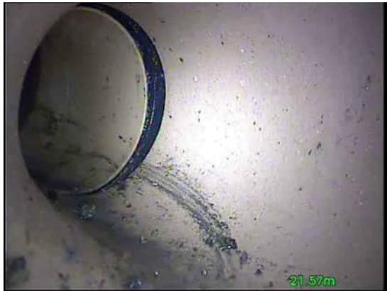
23, 00:02:27, 21.57 m Open joint, large
