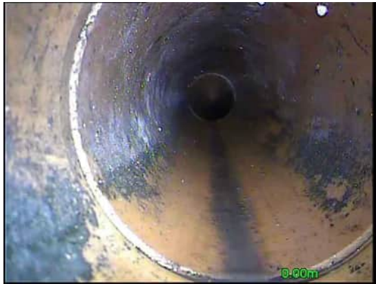
1, 00:00:03, 0.00 m Line deviates up
