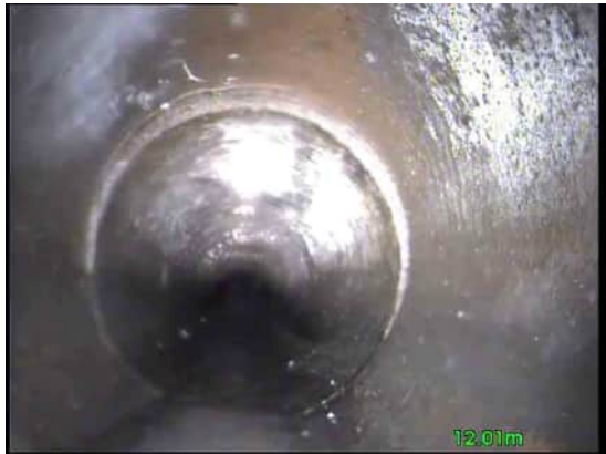
4, 00:02:54, 12.01 m Pipe material changes to cast iron at this point
