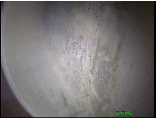
6, 00:00:36, 5.51 m Finish node, other special chamber, reference: RWP, RWP reached
