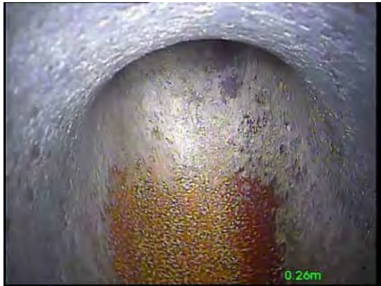
2, 00:00:07, 0.26 m Finish node, other special chamber, reference: Downpipe, Downpipe reached
