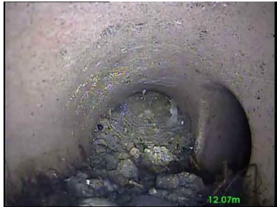
8, 00:00:49, 12.07 m Junction at 3 o'clock, 100mm dia
