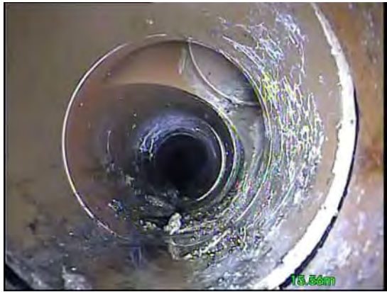
15, 00:01:52, 15.56 m Junction at 2 o'clock, 100mm dia
