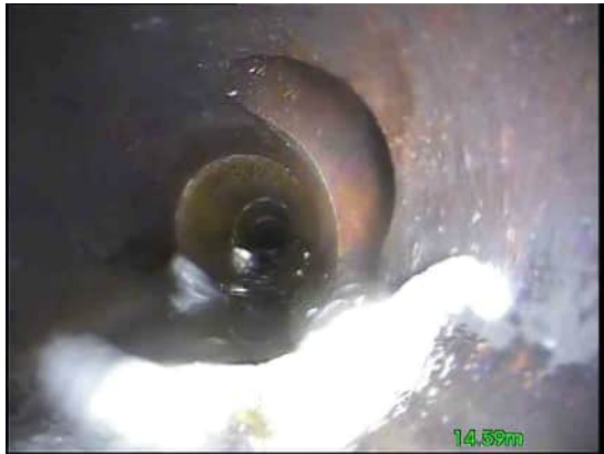
7, 00:01:07, 14.59 m Junction at 2 o'clock, 100mm dia
