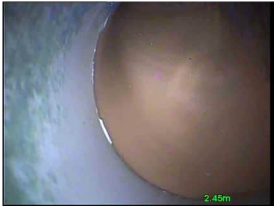
5, 00:00:15, 2.45 m Finish node, other special chamber, reference: Downpipe, Internal downpipe reached
