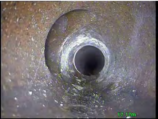
18, 00:02:06, 17.17 m Junction at 10 o'clock, 100mm dia
