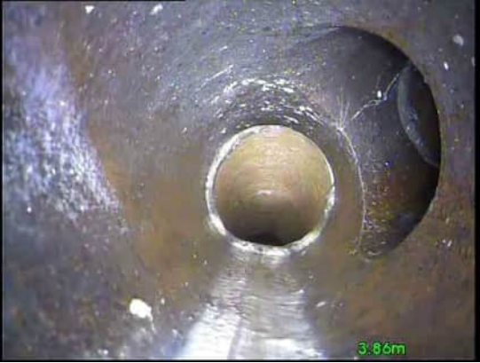
3, 00:00:17, 3.86 m Junction at 2 o'clock, 100mm dia
