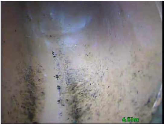
7, 00:00:54, 6.51 m Finish node, other special chamber, reference: Downpipe, Internal downpipe reached
