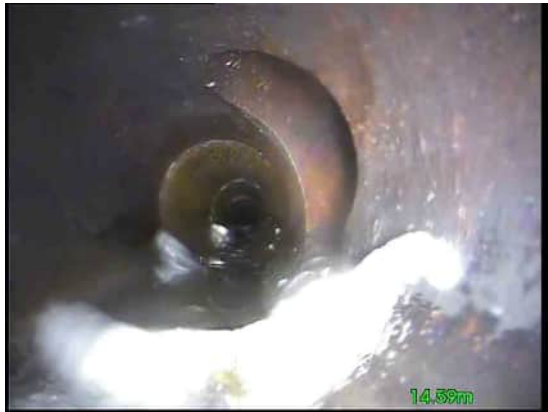
6, 00:01:07, 14.59 m Attached deposits, fouling from 4 o'clock to 8 o'clock, 10% cross-sectional area loss, start
