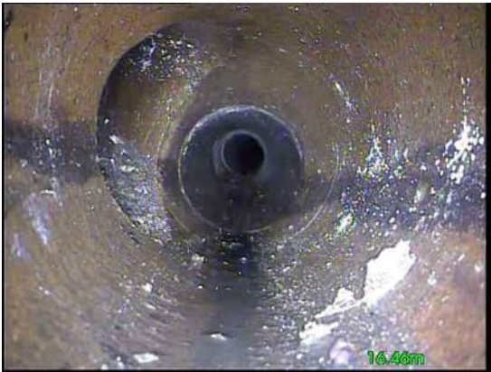
17, 00:02:00, 16.46 m Junction at 10 o'clock, 100mm dia
