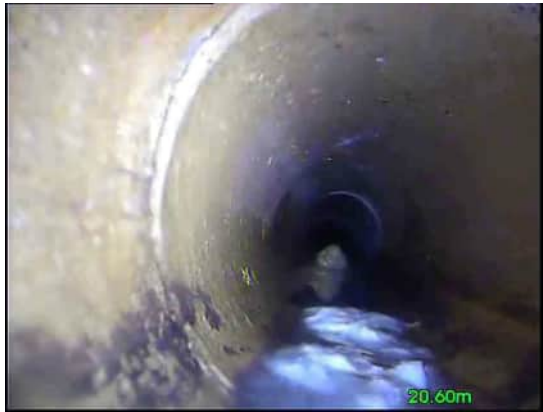
9, 00:01:45, 20.60 m Attached deposits, fouling from 5 o'clock to 7 o'clock, 5% cross-sectional area loss, start
