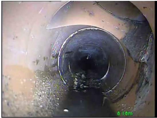
7, 00:00:54, 8.18 m Junction at 2 o'clock, 100mm dia
