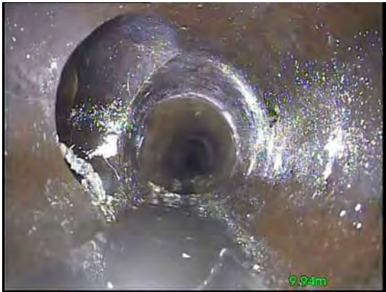
10, 00:01:09, 9.94 m Junction at 10 o'clock, 100mm dia
