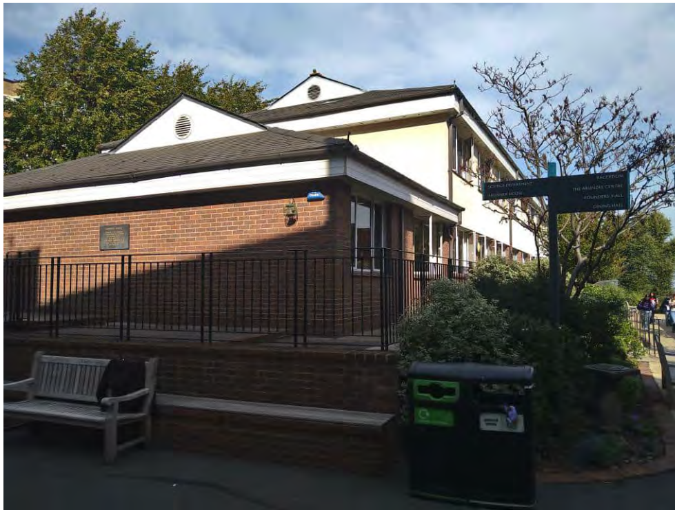
Image 1: Southern site boundary, viewing north
