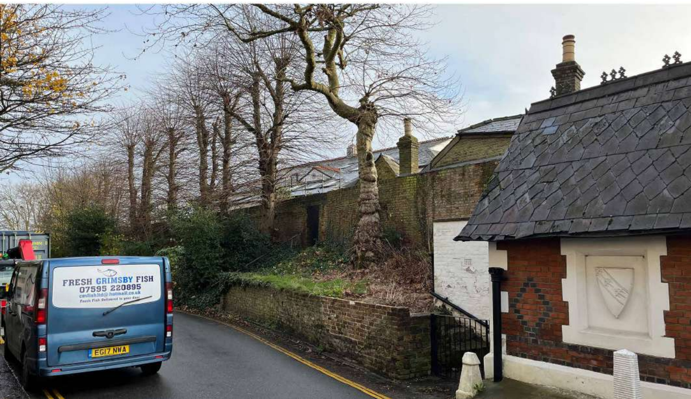
Fig 39. Existing view from Cholmeley Park, facing north
