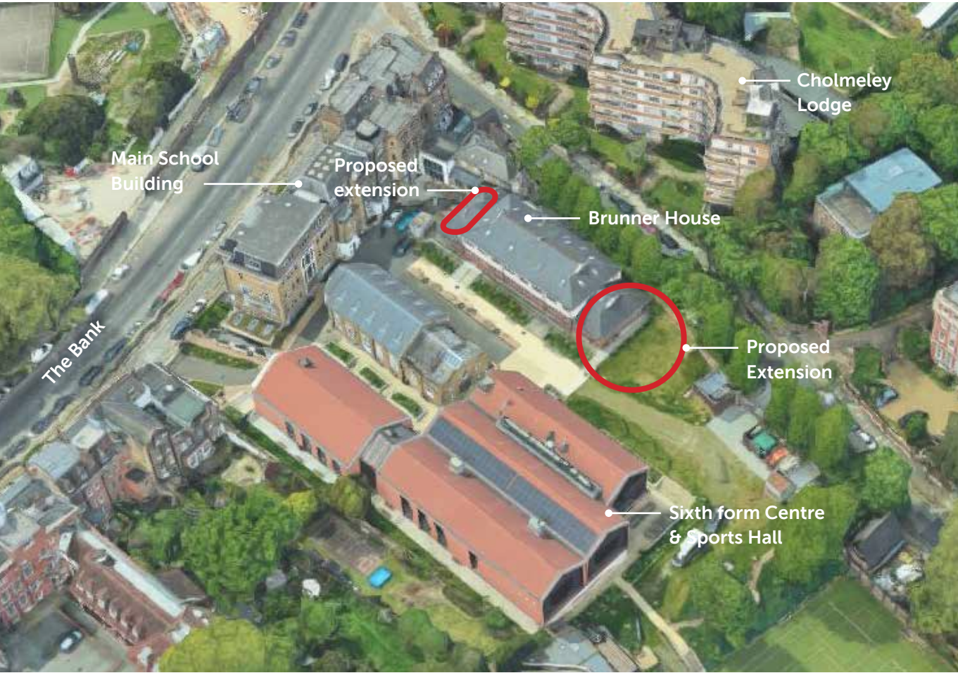
Fig 1. Aerial view looking east showing the location of proposed works.
