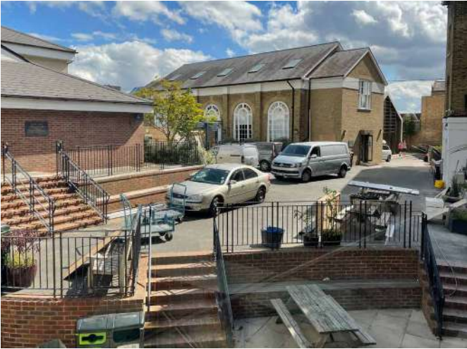
Fig 9. View of southwest elevation of Brunner House and outside space.
