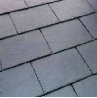
Fig. 29. Grey slate roof
