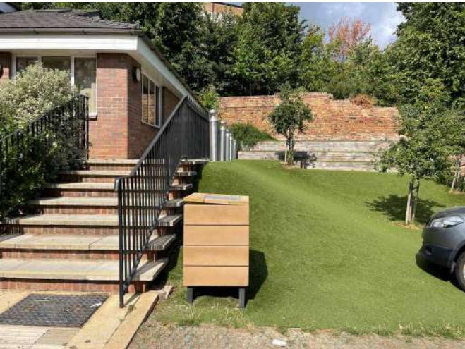
Fig 12. View of significant level change at the north-eastern end of the building.
