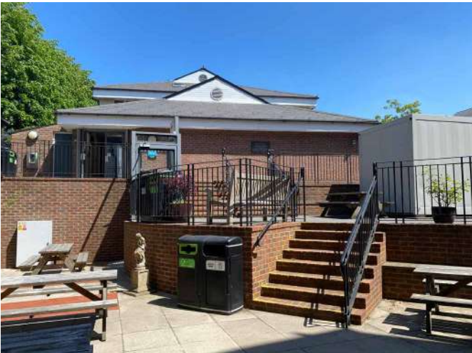
Fig 5. View of external platform lift enabling access to the front entrance of Brunner House.
