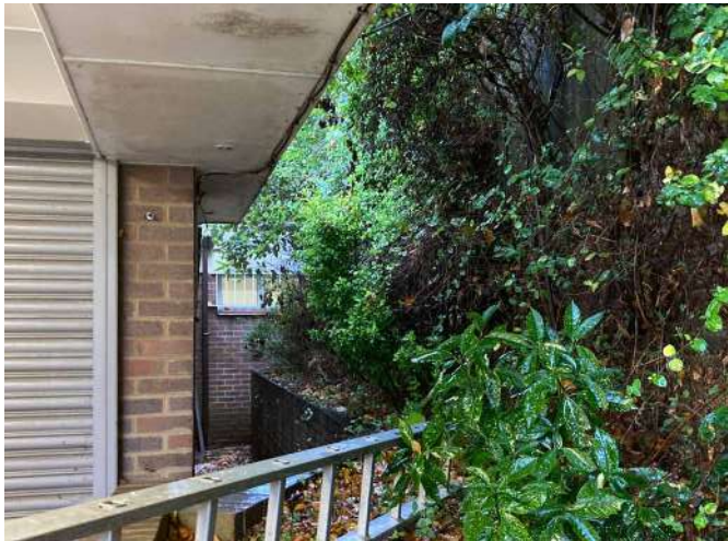
Fig 15. View of northwest elevation against boundary wall
