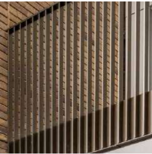
Fig. 33. Coated aluminium railings
