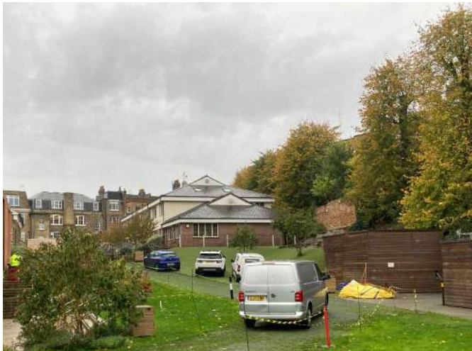
Fig 13. View of northeastern elevation of Brunner House.
