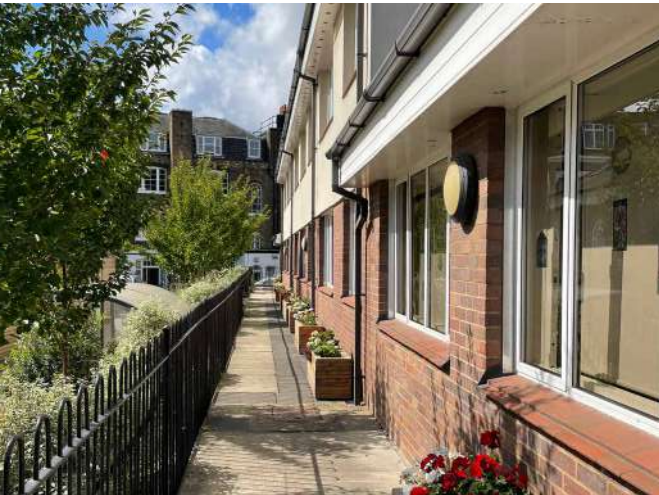
Fig 10. View of primary elevation of Brunner House.
