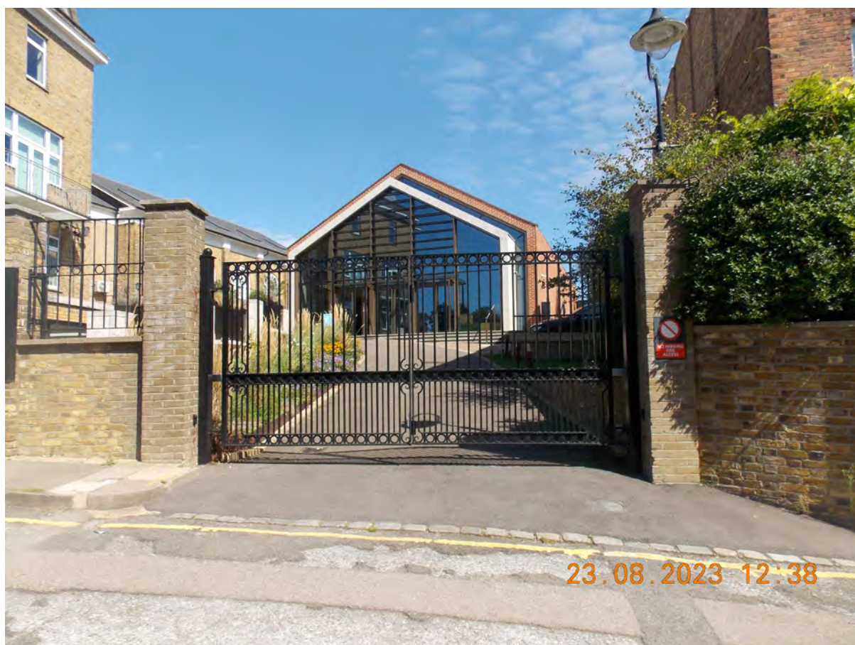
Fig 17. Photo of the modern building at the southern end of the site.
