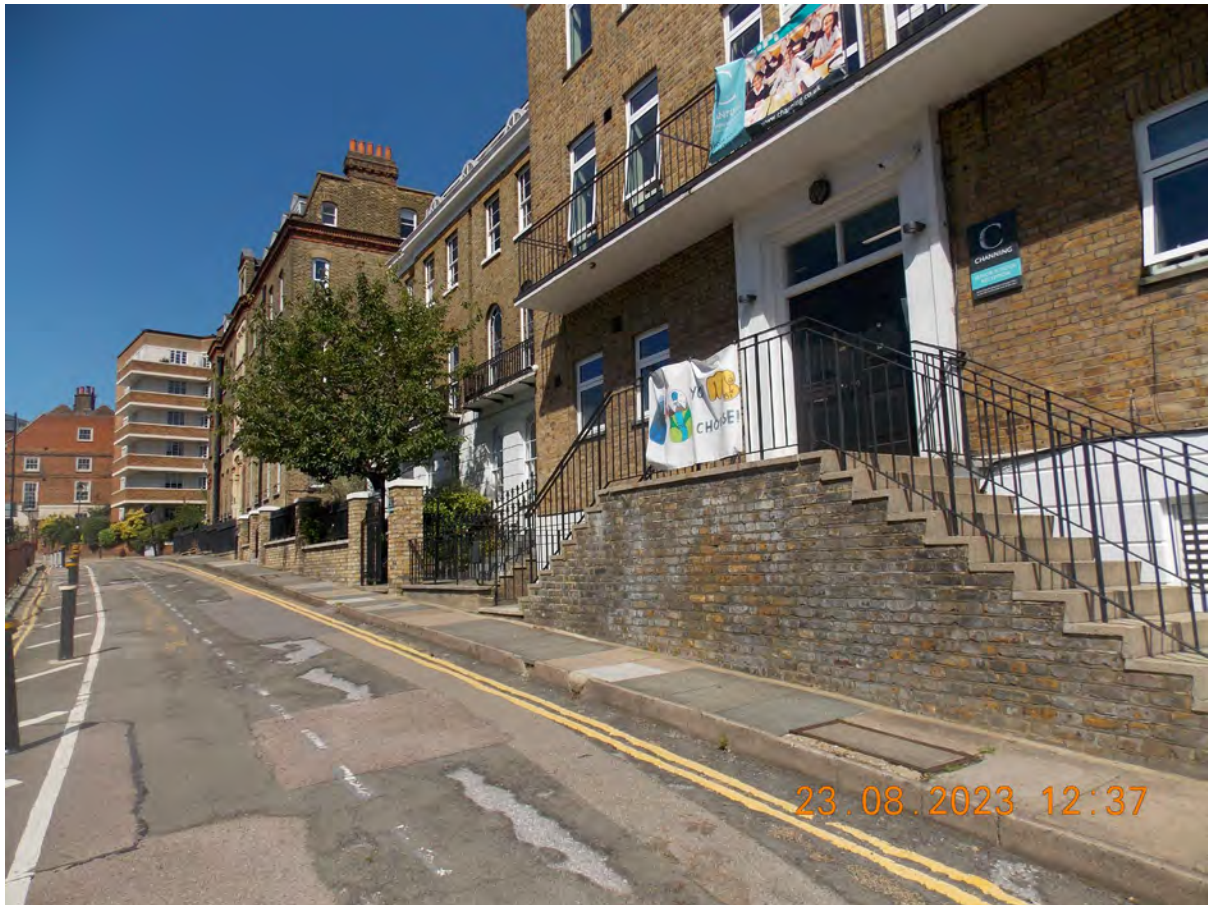
Fig 16. Photo of the main building on Highgate Hill looking north
