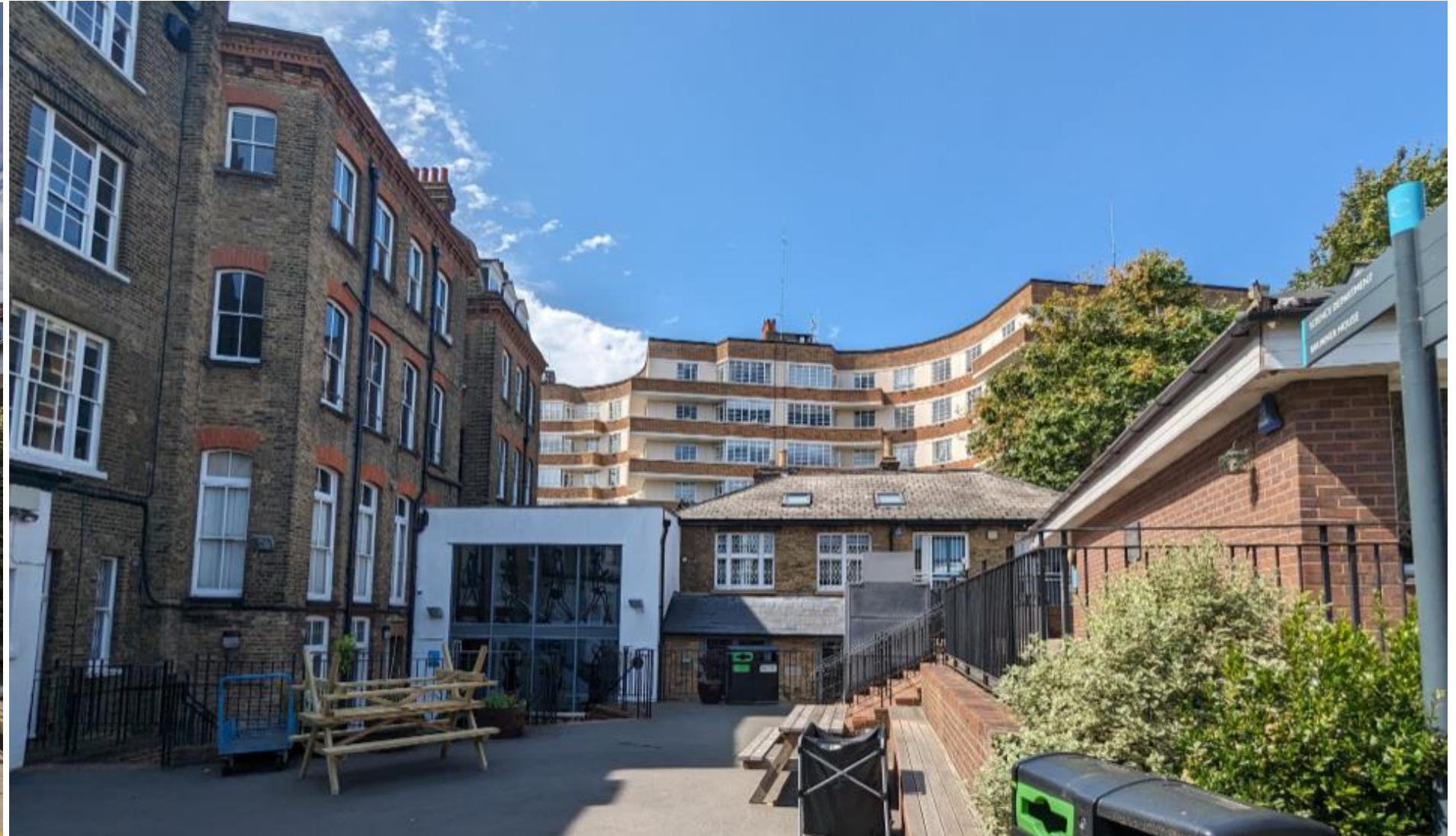
Figure 16: Juxtaposition between the Rear of Slingley & Westview and Brunner House (overlooked by Cholmeley Lodge)
