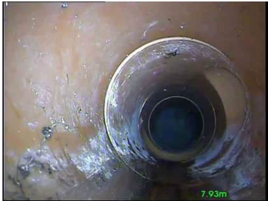
3, 00:00:30, 7.93 m Junction at 3 o'clock, 100mm dia
