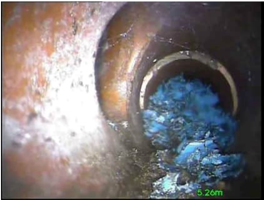
5, 00:00:30, 5.26 m Junction at 10 o'clock, 100mm dia
