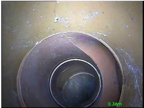
1, 00:00:09, 0.36 m Junction at 3 o'clock, 100mm dia
