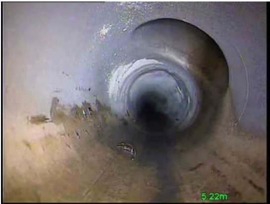
2, 00:00:24, 5.22 m Junction at 2 o'clock, 100mm dia
