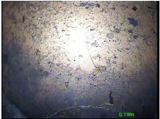
2, 00:00:08, 0.19 m Finish node, gully, reference: Buried Gly reached
