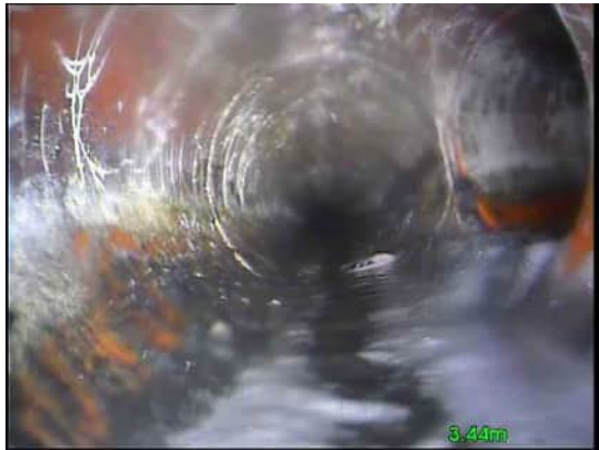
3, 00:01:53, 3.44 m Junction at 3 o'clock, 100mm dia
