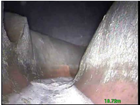
9, 00:01:01, 18.72 m Finish node, manhole, reference: MH31 UTL reached
