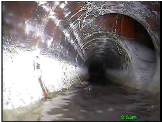
2, 00:00:17, 2.53 m Junction at 2 o'clock, 100mm dia
