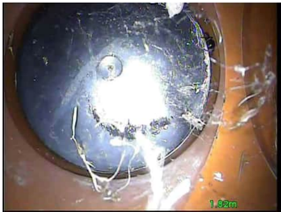
5, 00:00:27, 1.82 m Finish node, other special chamber, reference: Capped, Capped pipe reached
