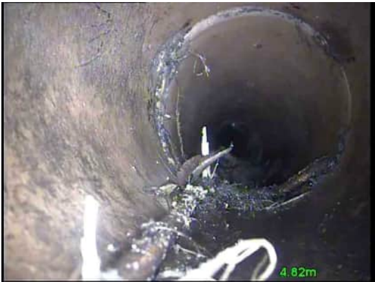
8, 00:00:45, 4.82 m Roots, mass, 20% cross-sectional area loss, start
