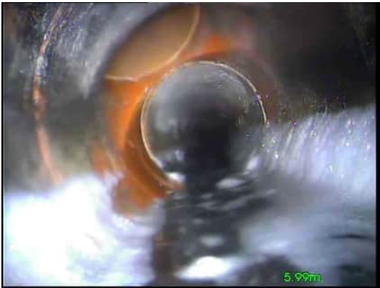
5, 00:01:37, 5.99 m Junction at 10 o'clock, 100mm dia
