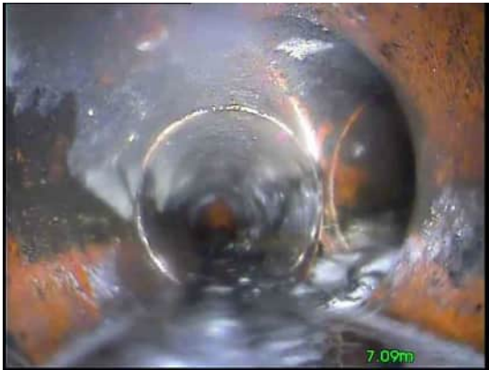
6, 00:01:31, 7.09 m Junction at 9 o'clock, 100mm dia
