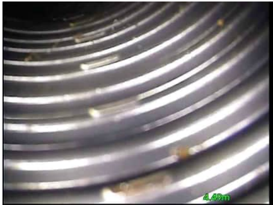
5, 00:00:40, 4.49 m Finish node, gully, reference: SGY reached
