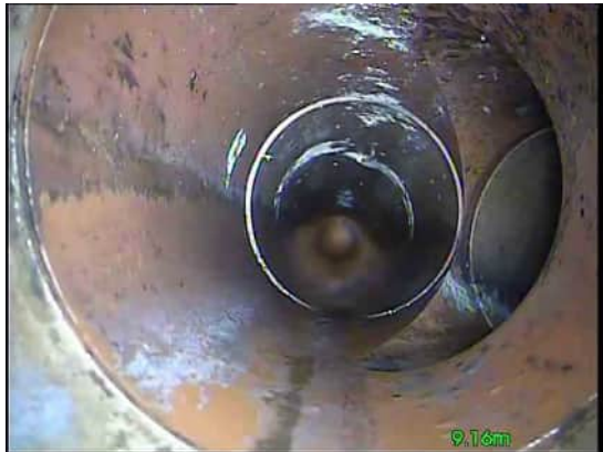
5, 00:00:41, 9.16 m Junction at 3 o'clock, 100mm dia
