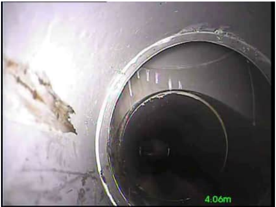
6, 00:00:34, 4.06 m Junction at 11 o'clock, 100mm dia
