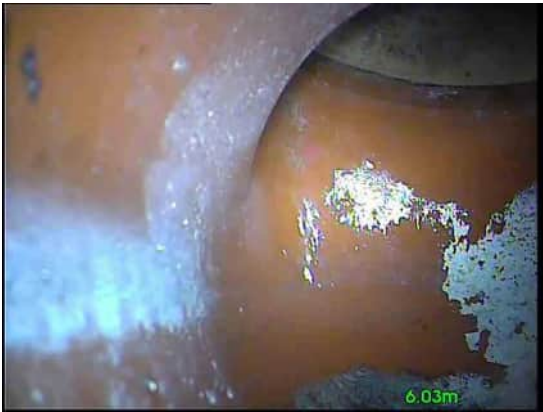
5, 00:00:42, 6.03 m Finish node, other special chamber, reference: Downpipe, Internal downpipe reached
