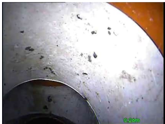
2, 00:00:05, 0.26 m Junction at 12 o'clock, 100mm dia
