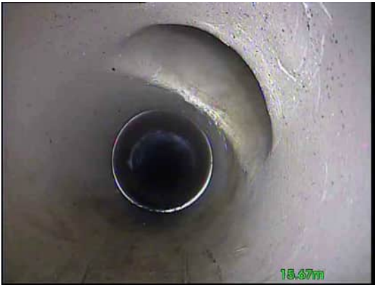
5, 00:01:01, 15.67 m Junction at 2 o'clock, 100mm dia
