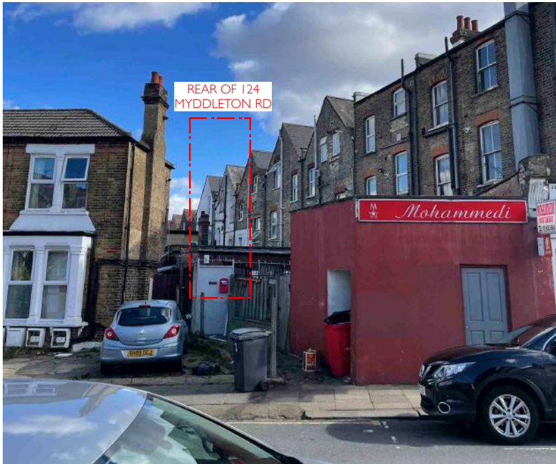
B SIDE VIEW OF THE REAR OF SITE FROM WHITTINGTON RD
