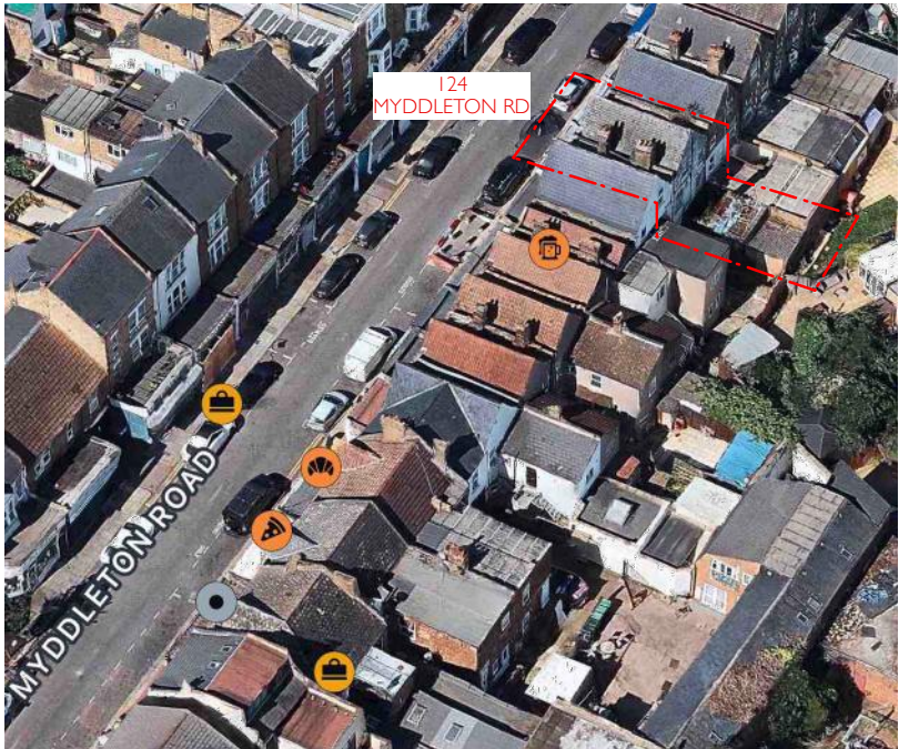
C AERIAL VIEW LOOKING TOWARDS THE REAR OF SITE
