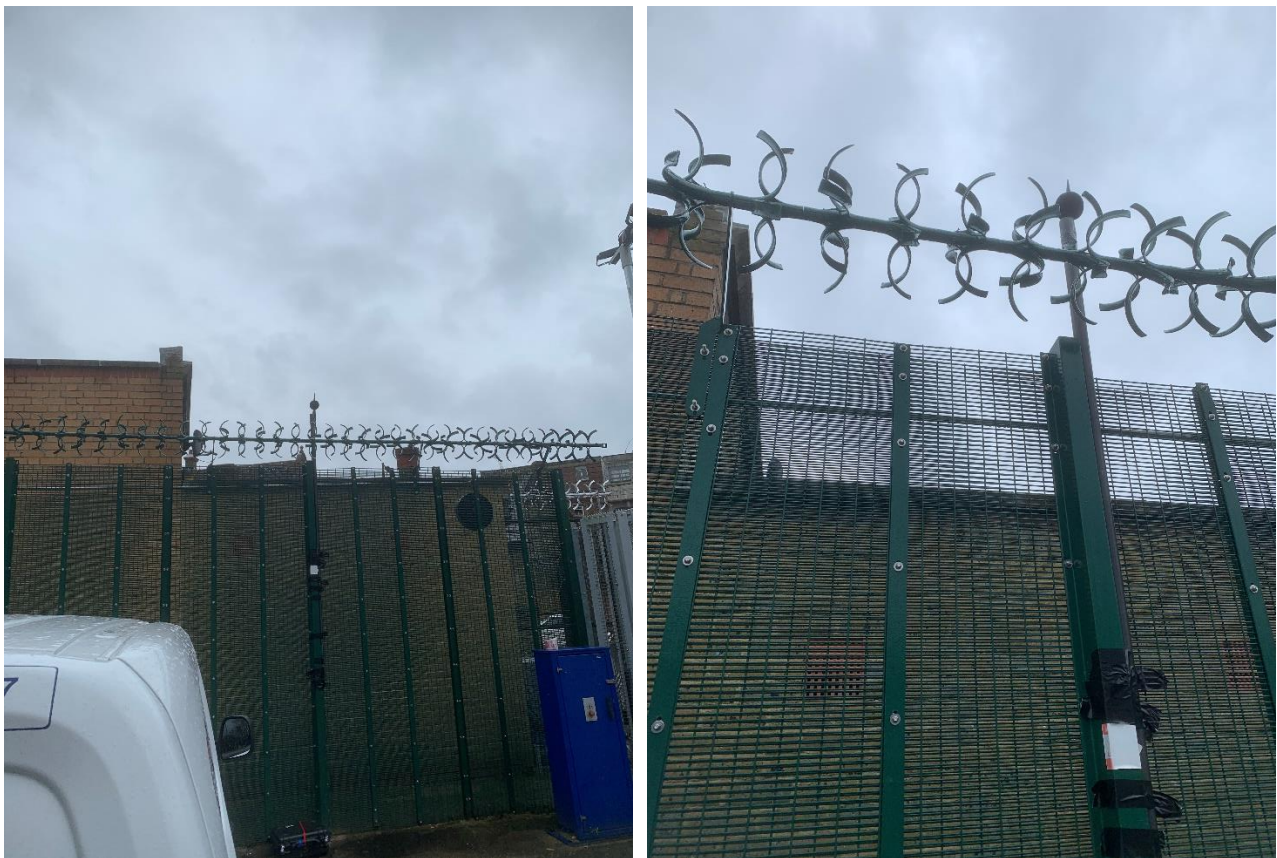
Figure A.3.2 Fixed measurement location in situ
