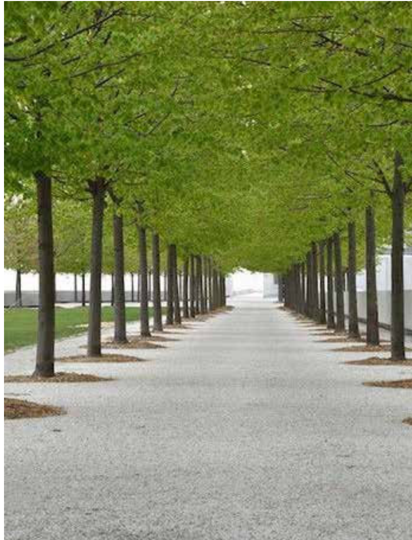
Example of self-binding gravel
