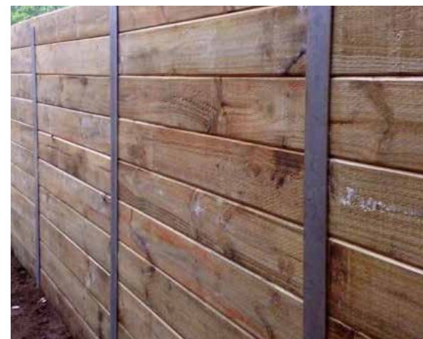
Reinforced hardwood sleeper retaining wall
