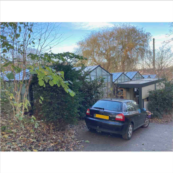
East Elevation from Access Road
