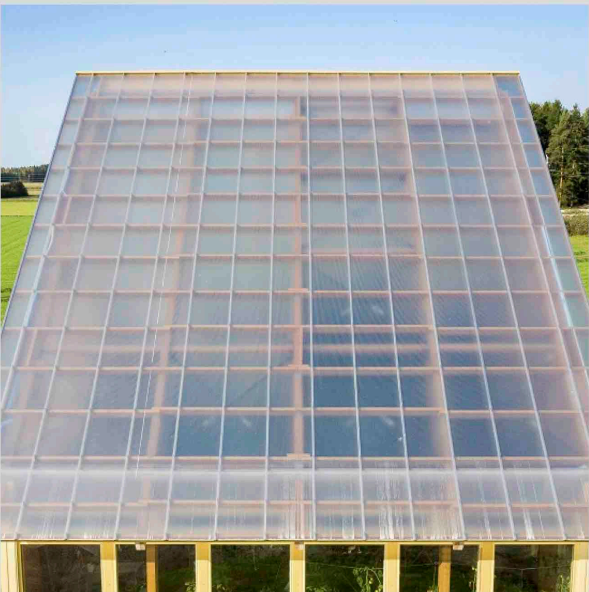
Walls/Roofs - Translucent/obscured multi-wall polycarbonate cladding/roofing.
