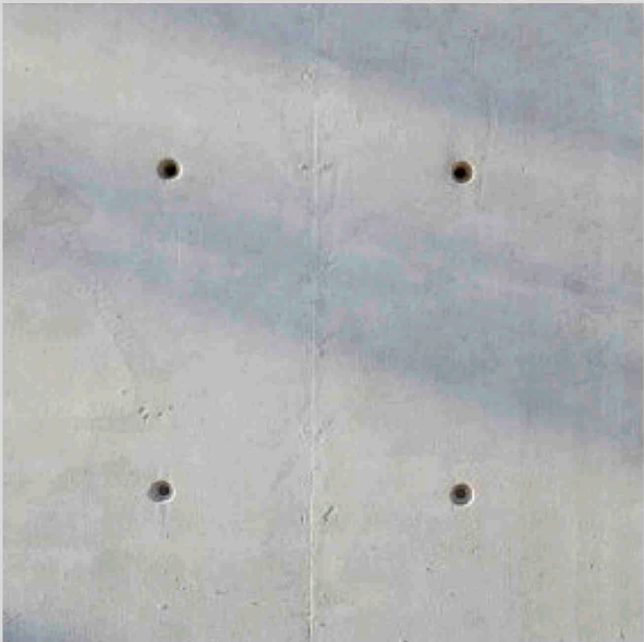
Retaining Walls - Fairfaced concrete retaining walls
