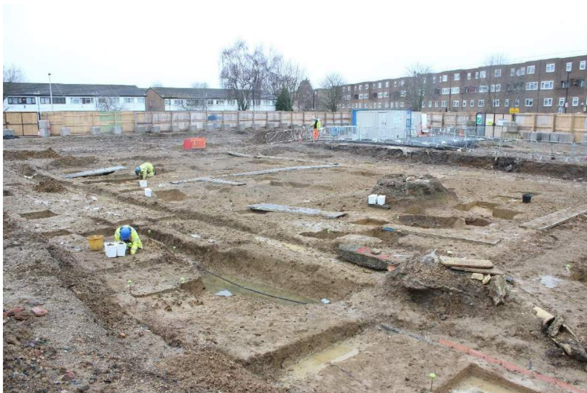
Plate 5: Working shot, southern half of site looking north-west: grid square excavation following clearance of modern service trenches and archaeological features.
