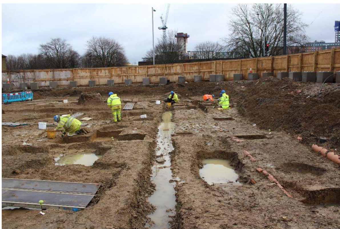
Plate 6: Working shot, southern half of site looking east: commencing work on grid squares in area of Scatter B following clearance of modern services and archaeological features.
