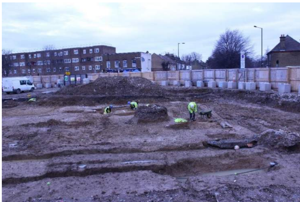
Plate 3: Working shot looking north: excavation of medieval features.
