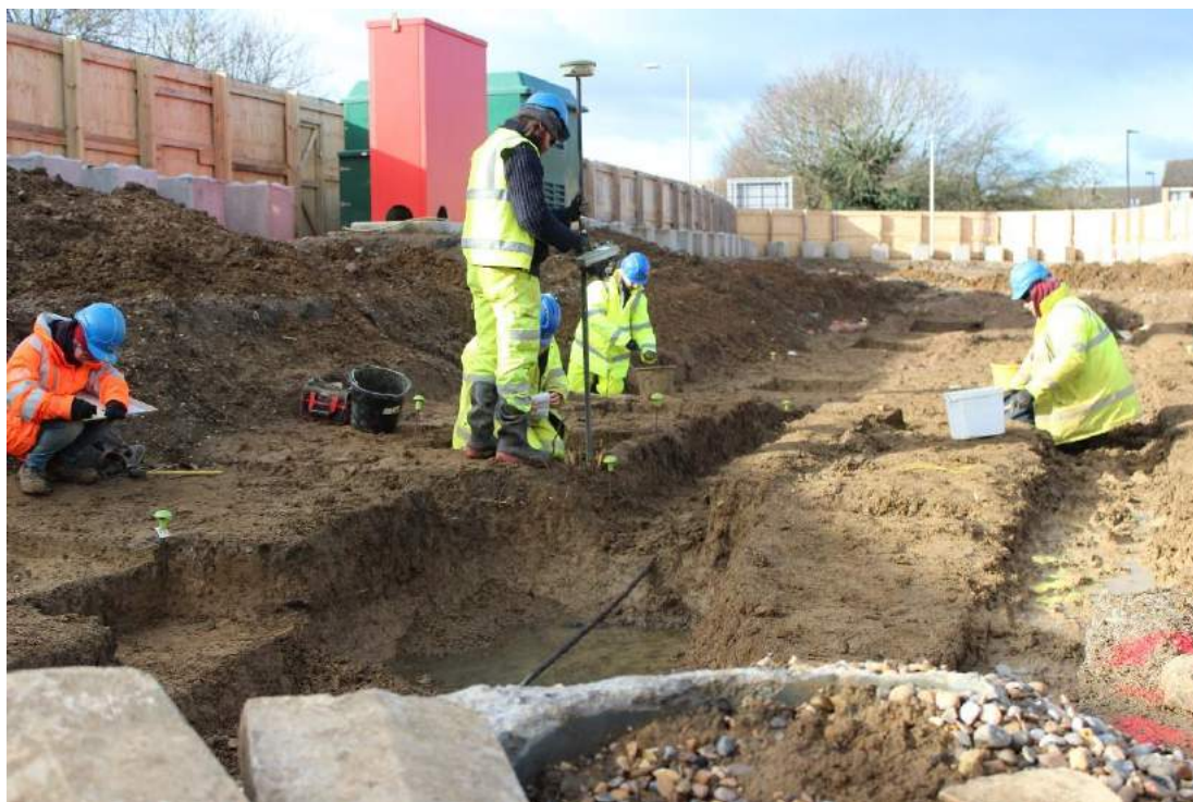
Plate 8: Working shot, excavation/recording and logging lithic locations.
