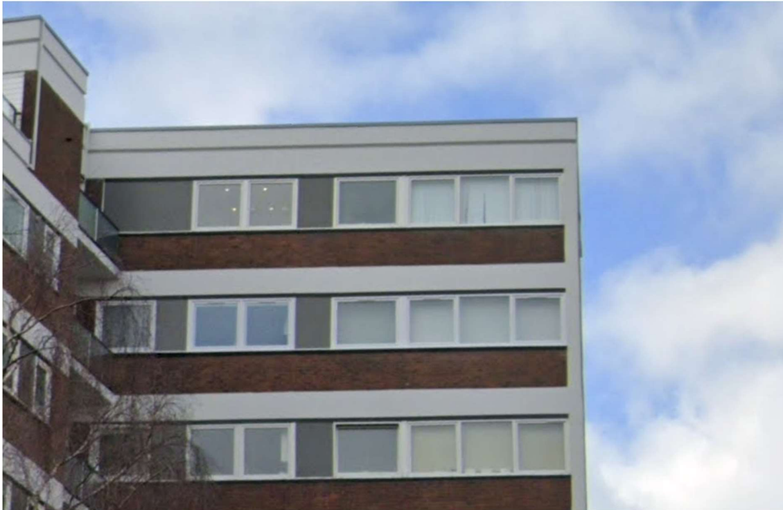
Figure 2 – High Sheldon – View taken from street looking at the neighbouring block where the window fenestration for the top floor flat mimics the design below.
