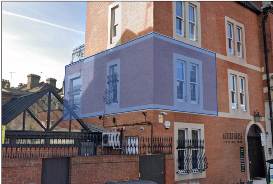
Figure 4: 6.2 Hubert House Mezzanine Studio
