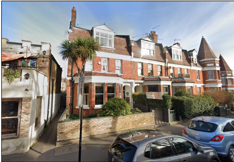
Figure 6: Properties north of Weston Park
