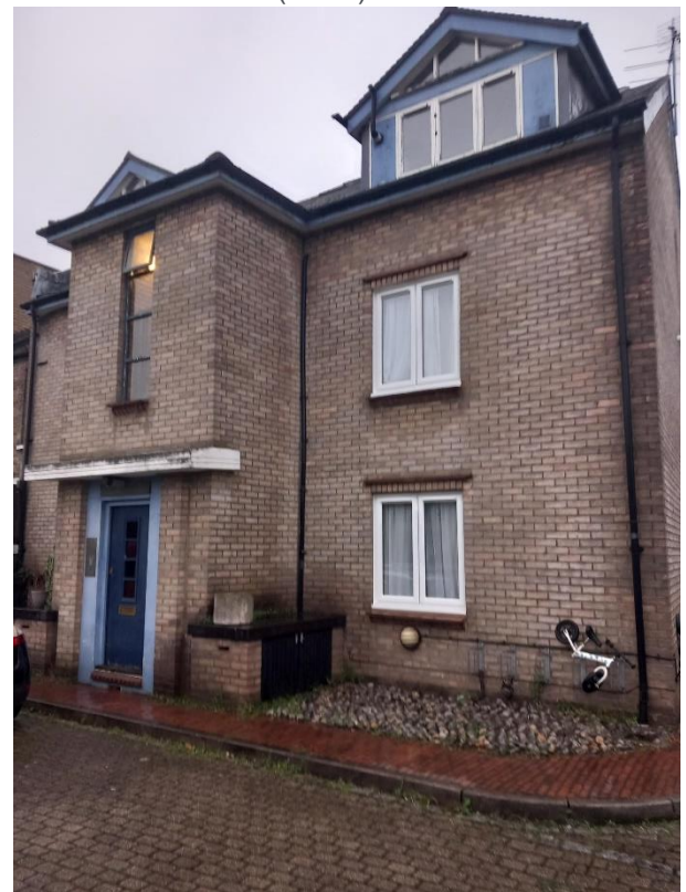
Context view of block entrance door
