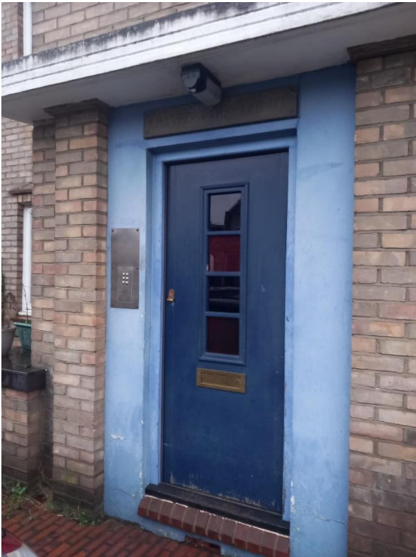
Block Entrance Door
