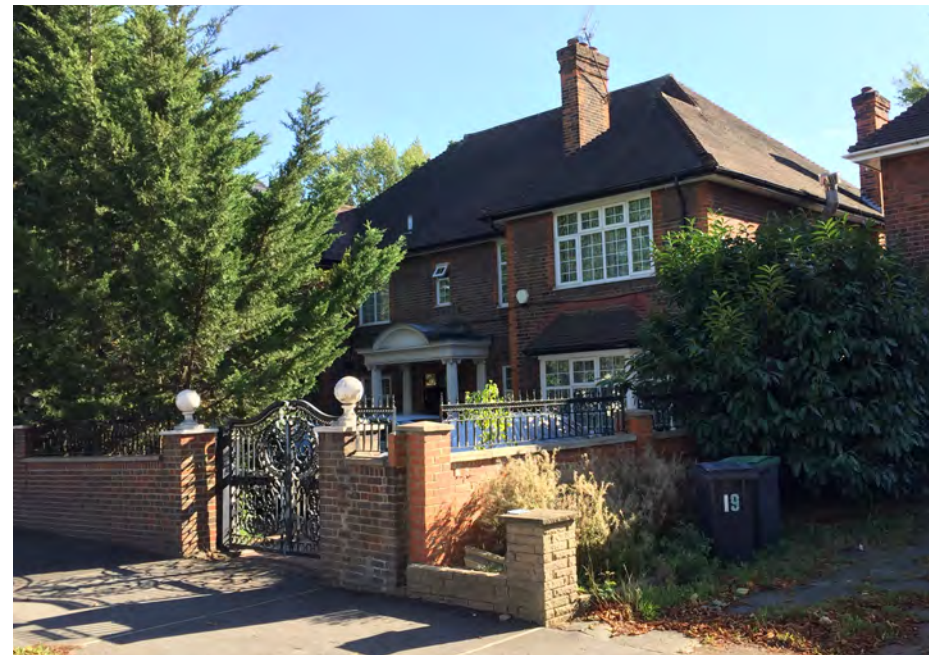
21 Aylmer Road Nos. 23, 21, 19 and 17 Aylmer Road appear to have been built to the same original design. Of the four houses no.21 seems to be the one that remains closest to the original form and appearance. It can be described as an Arts and Crafts style house, with symmetrical frontage with a classical columned porch. There is some brick detailing at the external corners and window openings that gives a sense of craftsmanship. UPVC framed windows have replaced the original windows.
