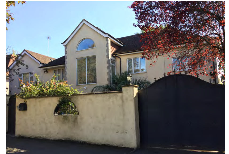
25 Aylmer Road is the immediate neighbour to the west of the subject house. Haringey Council granted consent for the house to be enlarged and altered by the addition of a large two-storey gabled front extension and a two-storey side extension on the east side under planning permission ref. HGY/2003/0049. The rendered walls are painted in an off-white cream colour and have false quoins on the external corners. The original main volume of the house has a hipped roof and the later additions have gabled roofs.
