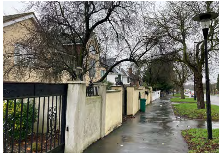
View along Aylmer Road looking west showing (from left to right) no.25, no.23 and no.21.
