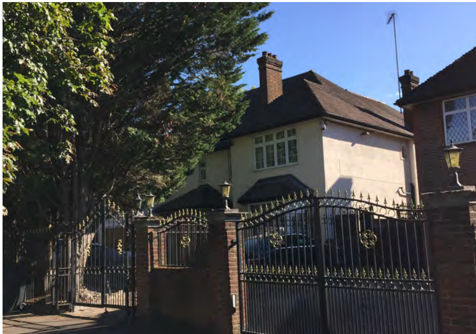
17 Aylmer Road has the same overall form and design as no 21 and was likely built at the same time. By contrast to no.21 the original brickwork has been rendered and painted cream. The porch has a hipped roof. The left-hand bay has an integrated garage at ground floor level and a single-storey extension has been added on the east side that fills in the gap between the side elevation and the party fence line.
