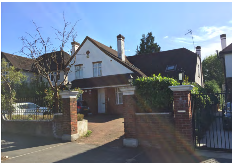
11 Aylmer Road appears to also be inspired by domestic Arts and Crafts architecture with a large asymmetrical gable on the left hand side and low eaves at the front. The brickwork detailing is simple but well crafted. Similar to the immediate neighbouring houses the ground floor is in brick with painted render above.
