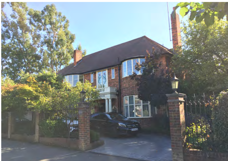
Wallbrook House (next to 1 Aylmer Road). The house has a character which can be described as Arts and Crafts, and the original composition appears symmetrical with a matching pair of two-storey curved bays set on either side of the entrance porch. The porch has classical columns supporting an entablature with balustraded parapet above. A two-storey extension appears to have been added at the east side, which has broken the original strict symmetry of the composition. (Note: Wallbrook House is outside the boundary of the Highgate Conservation Area.)
