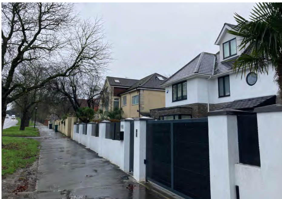
View along Aylmer Road looking east showing no.23 on the right in the foreground with no.25 to the left.
