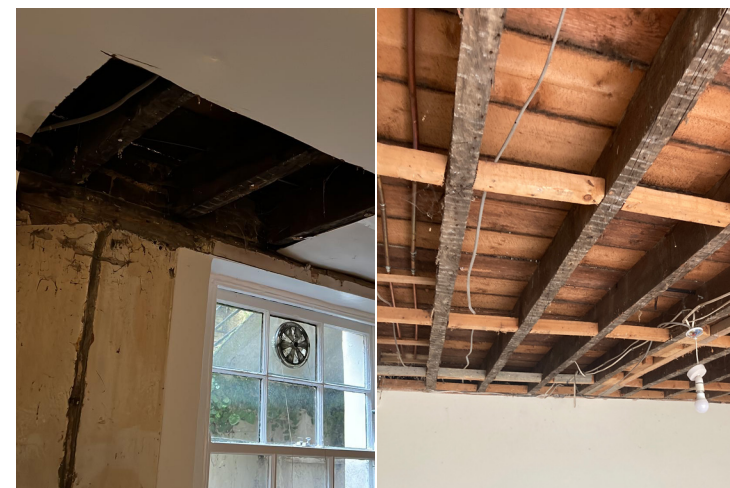
(1) Modern plaster board ceiling in the kitchen. (2) Modern noggin timber between historic joist.
