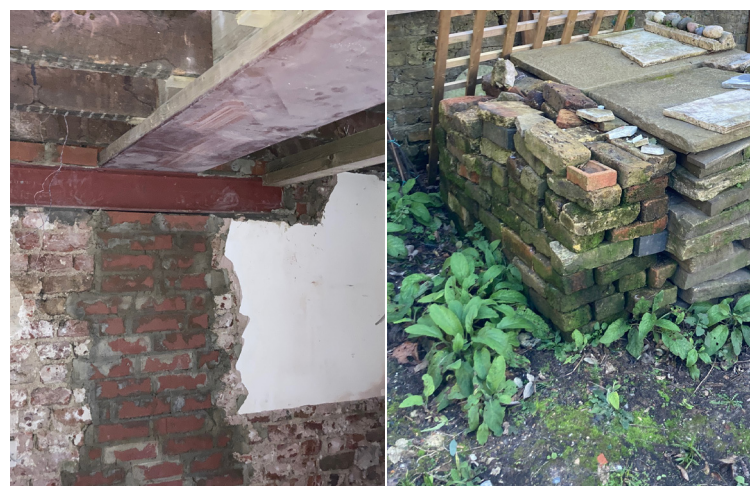
(1) New Steel inserted onto padstones in party wall. (3) Bricks to be reinstated
