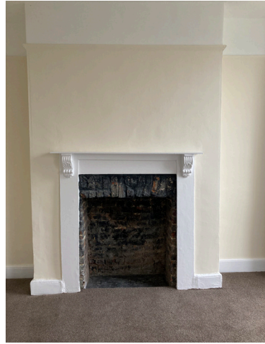
(1) Existing surround has been removed
