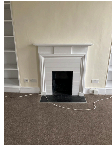
(1) Existing Fireplace, hearth & shelves.
