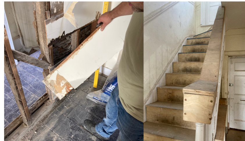
(1) Modern timber boarding cladding to the internal stud walls.
