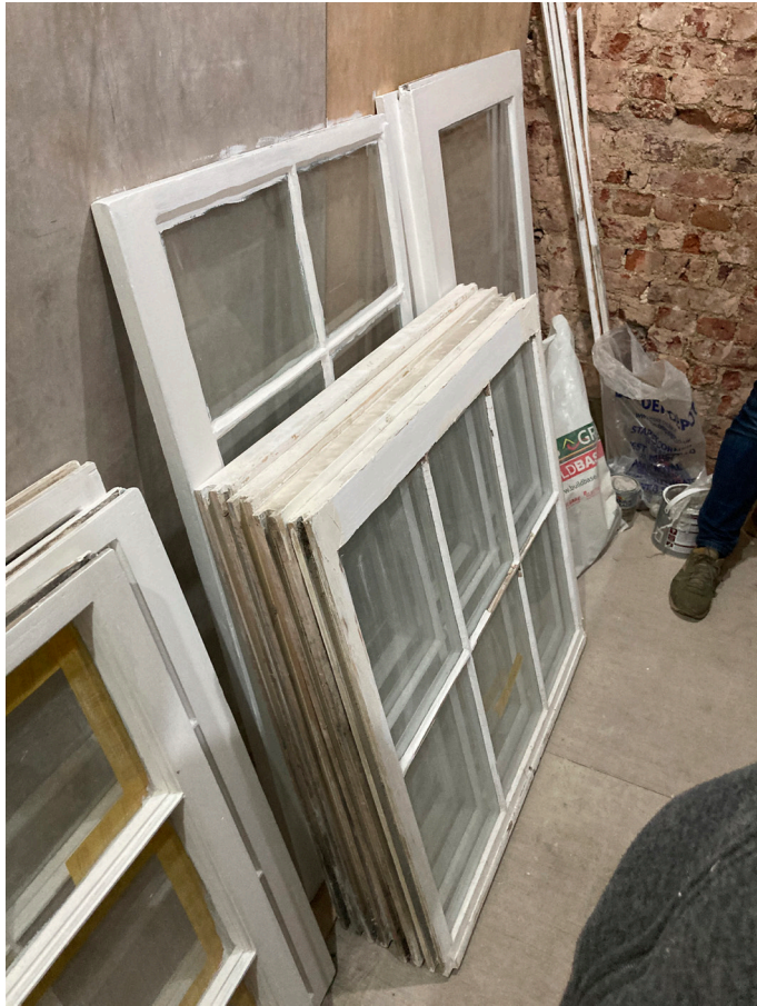
Existing windows have been removed and are on site for repair and making good.
